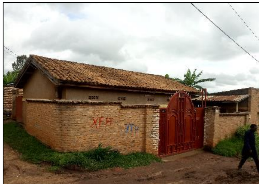
PAffected Household Structure – House & Fence on RoW
