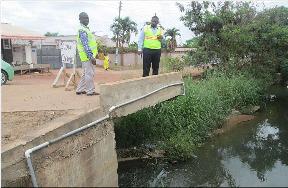
Plate 1-2: Site inspection at Dome –Kwabenya. (Third culvert)
