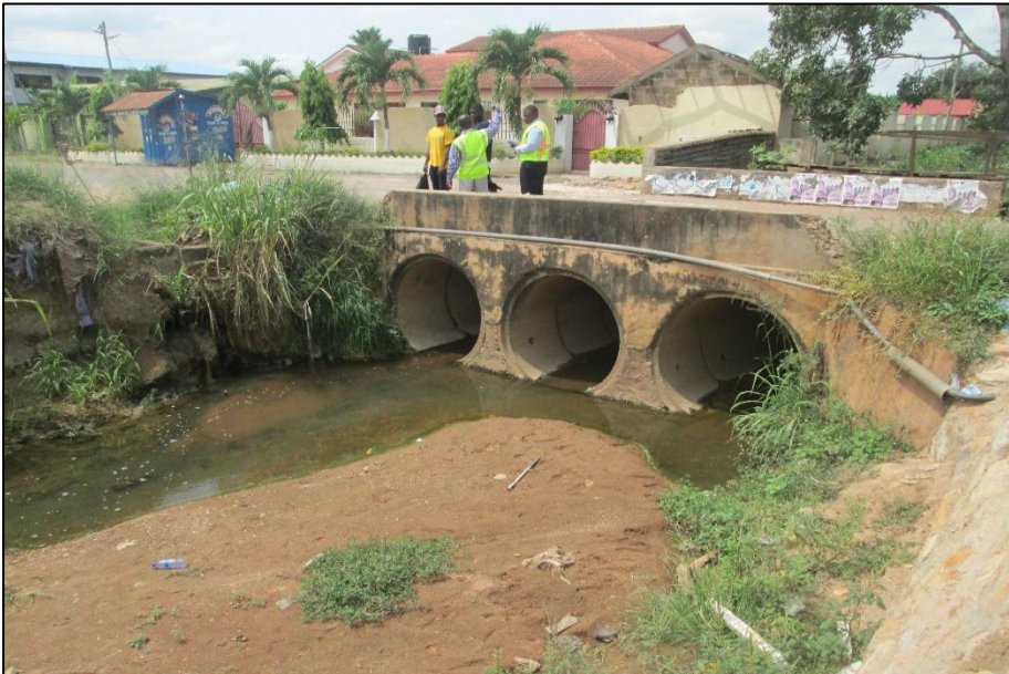
Plate 1-1: Site inspection at Dome –Kwabanya (First culvert)
