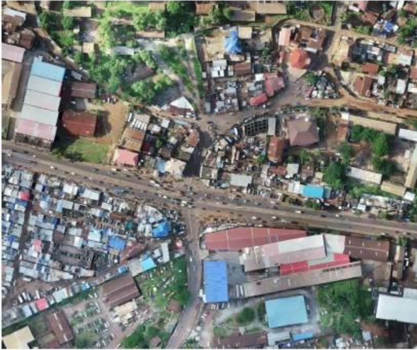
Figure 6.3-2: Aerial View of Kissy Ferry Junction Intersection. Source: MoTA
