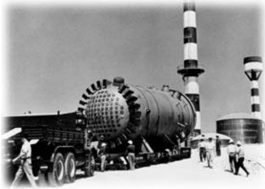
Boiling water reactor vessel arriving at the Garigliano site, December 1962. Photo: General Electric.
