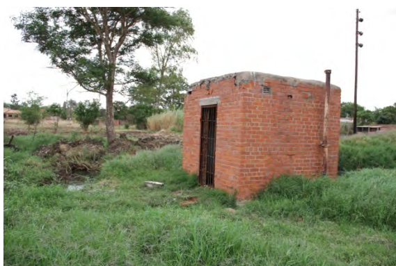
Tangatara Sewage Pumping Station
