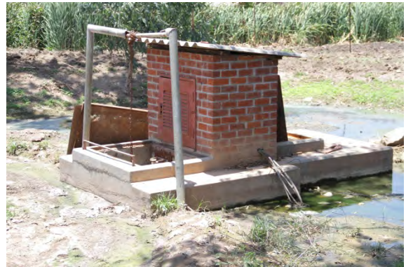
Relnyaro SPS: Wet well and superstructure
