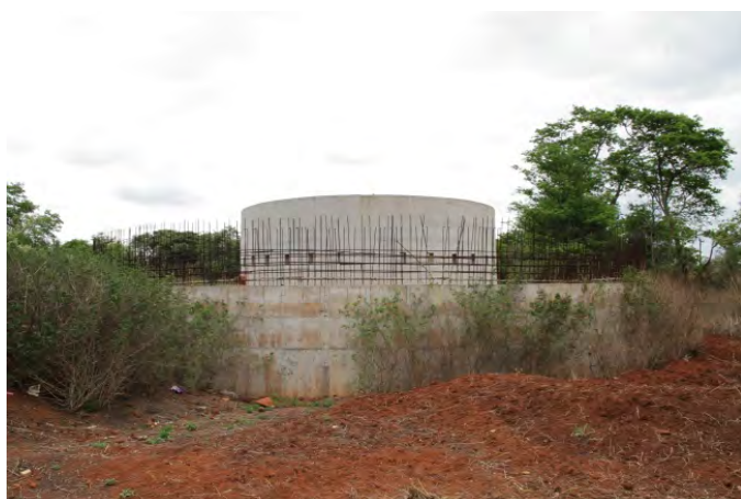
Partially Complete FC Reactor
