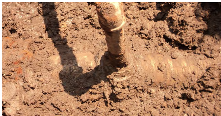
Asbestos Cement (AC) pipe
