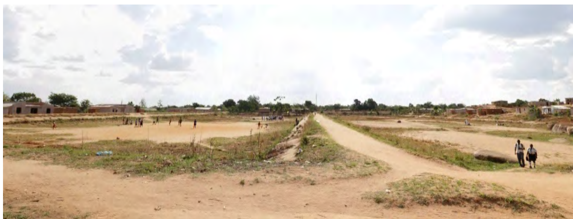
Epworth Sewage Ponds
