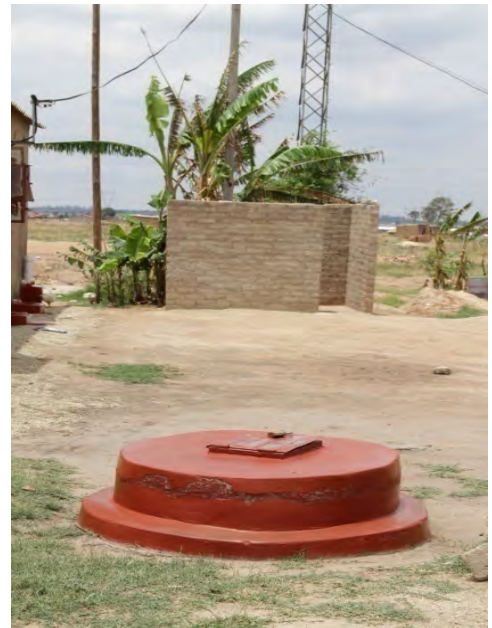
Well maintained private shallow well. Note the proximity of the shallow well (foreground) to the pit latrine (background)
