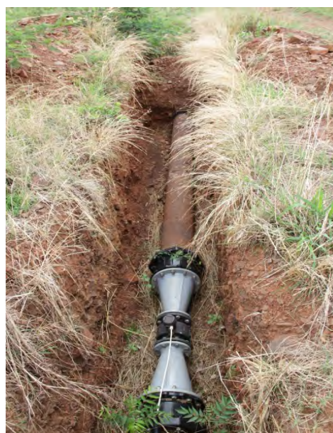
GIZ Installed Flow Meter into Norton Tanks
