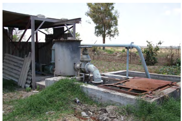
Chilemba SPS: Temporary Pumping Arrangement
