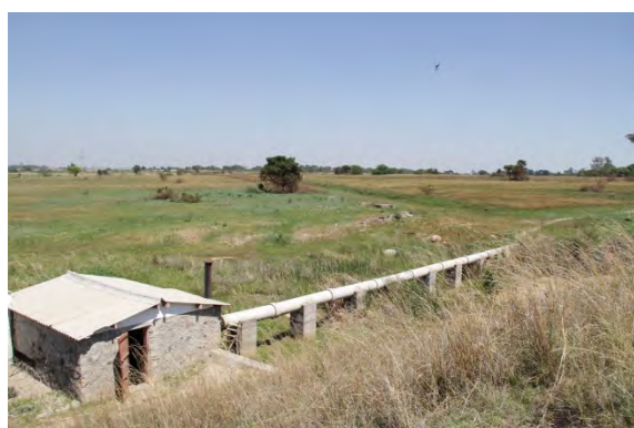
Green Sykes Raw Water Pump Station
