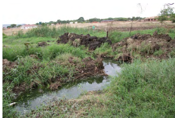
Sewage Overflow from Burst Force Main
