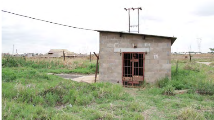
Maridale Sewage Pumping Station
