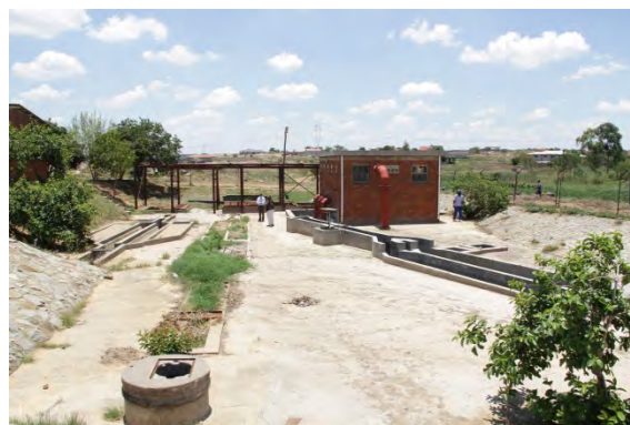
Ruwa Main SPS: Inlet works left and center to old wet wells and right to new station
