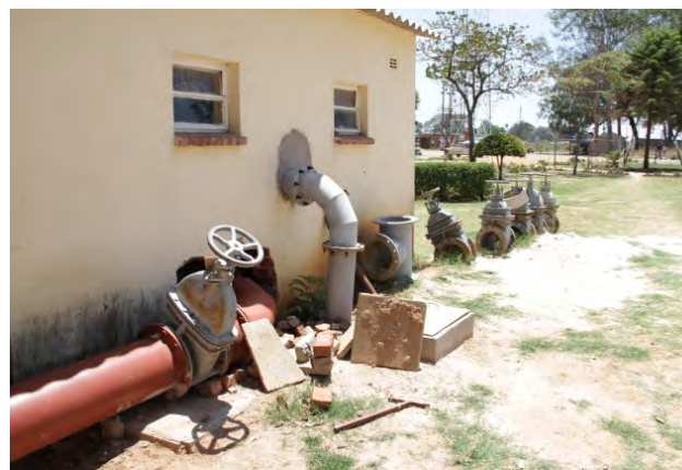
Mutare Road P/Stn: Works underway to new pumps to Damofalls
