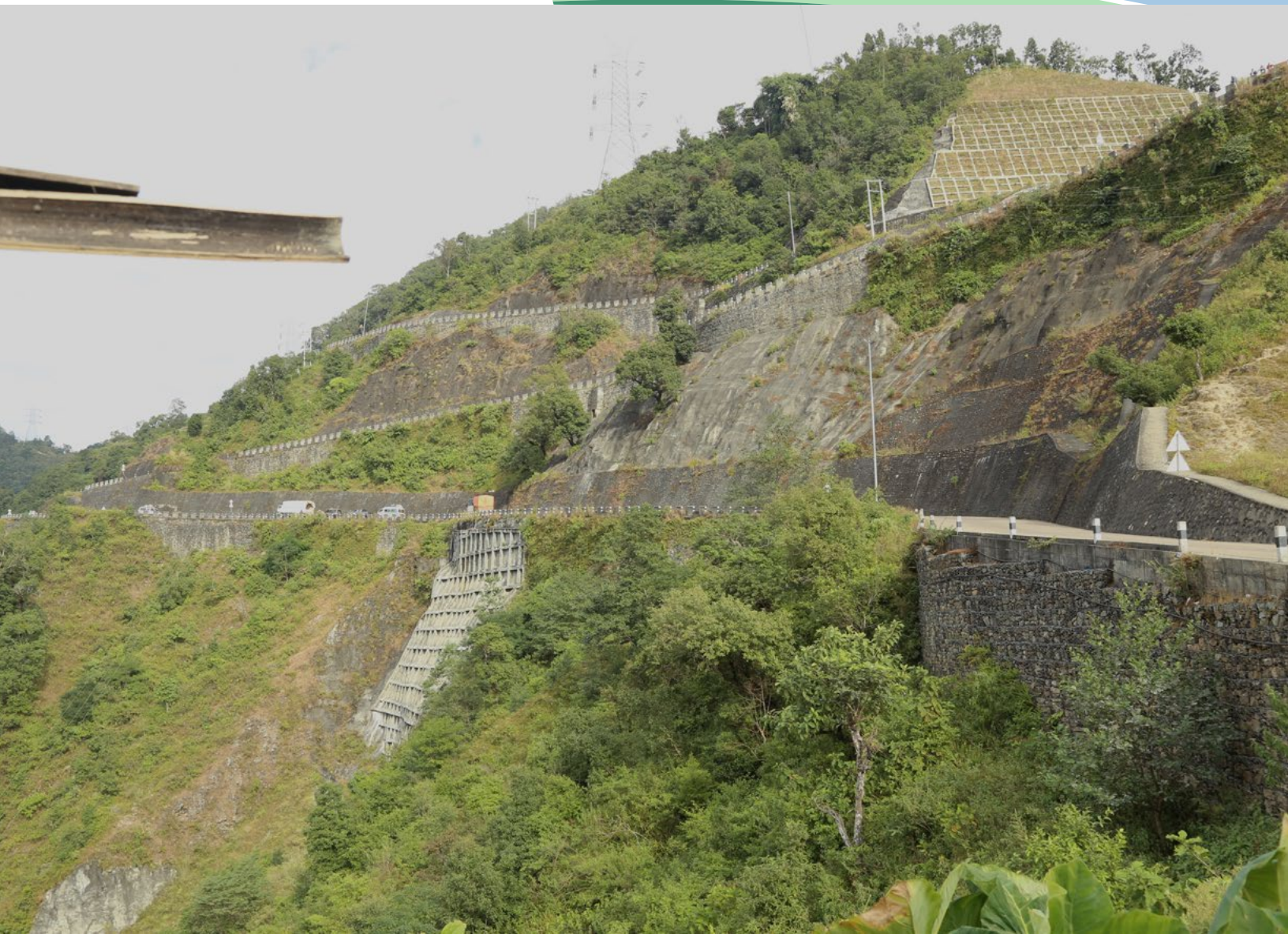
PLATE 5: Heavily-engineered design. Earth-reinforced walls; bolted reinforced concrete crib walls and shotcrete.
