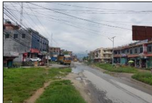
Road in Talchowk at starting Area
