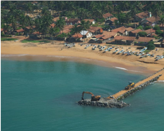
FIGURE - 20: HARD AND SOFT MARAWILA BEACH SAND NOURISHMENT FOR COASTAL PROTECTION
