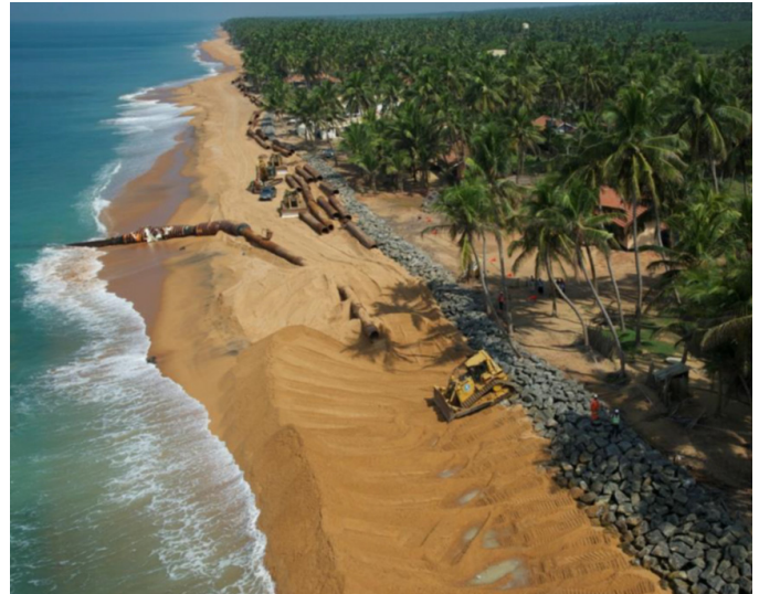
FIGURE - 20: HARD AND SOFT MARAWILA BEACH SAND NOURISHMENT FOR COASTAL PROTECTION
