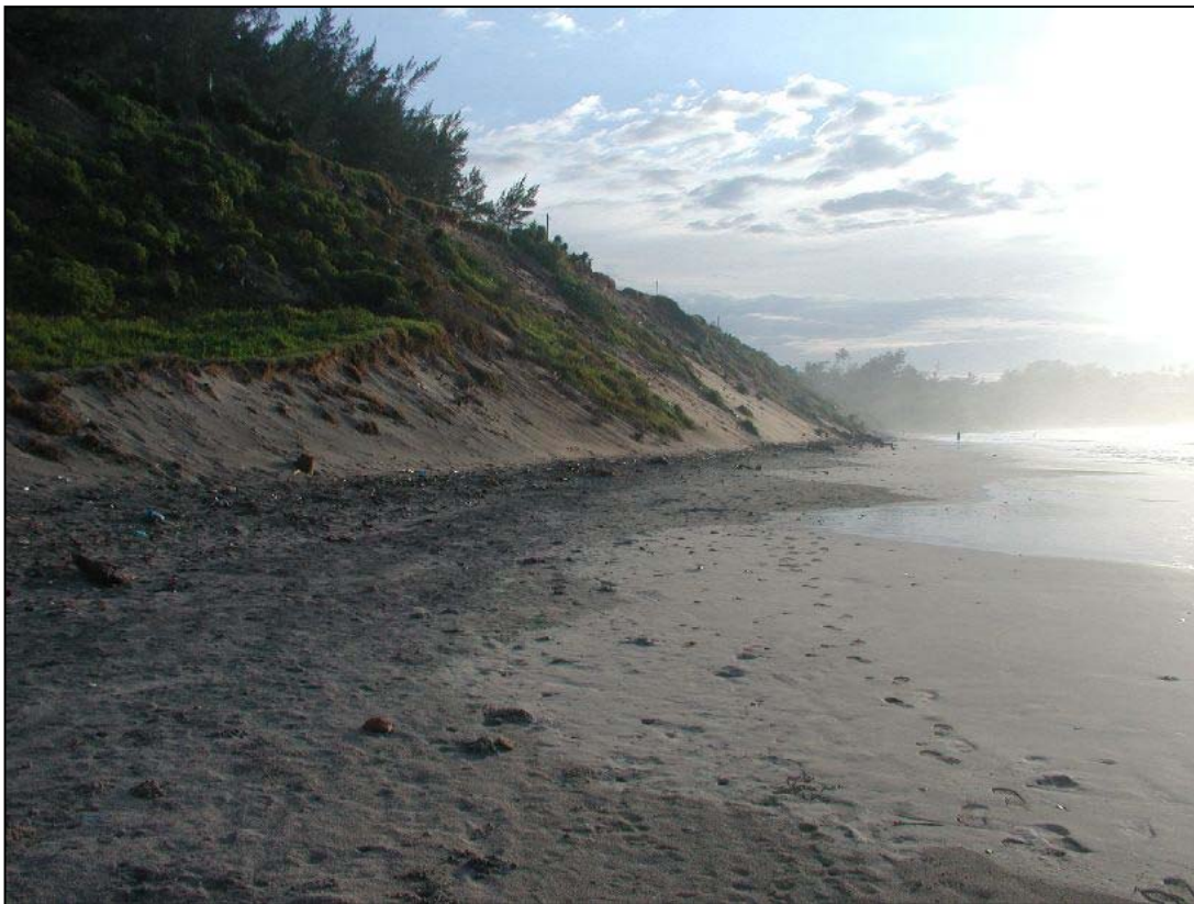
Figure 2.4 Coastal Road on Actively Eroding Bluff Near Fort Dauphin
