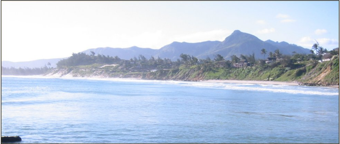
Figure 2.3 Shoreline Erosion at the North End of Fausse Baie des Galions
