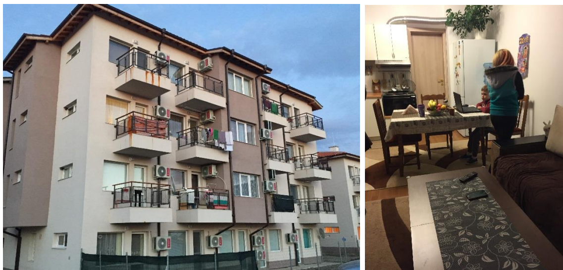
Plate 8.3 New Social housing project in Dupnitsa
