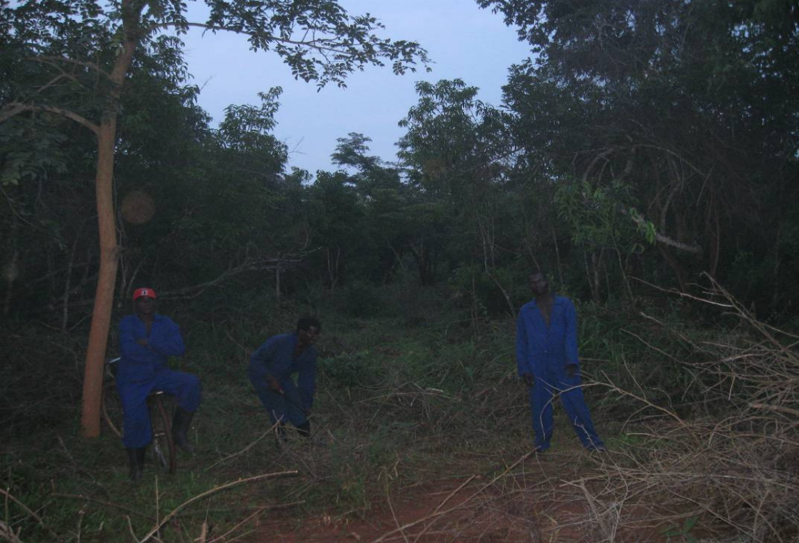
Figure 14: Photo of Workers at Work
