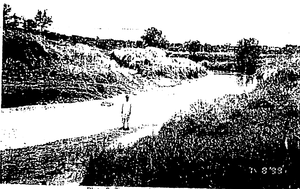
Plate 8 Torrent with stabilized banks
