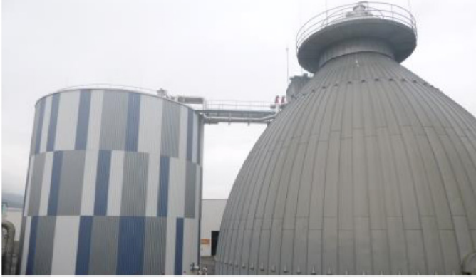
CS #1: Heated sludge digesters of different shapes (Europe), used for digesting sludge from CAS
