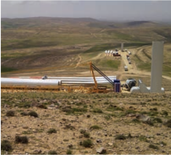
Wind power project in the construction phase
