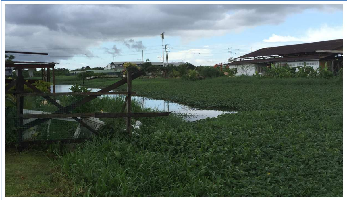
Figure 3-8. Saramacca Canal towards more rural western end, showing weed growth.
