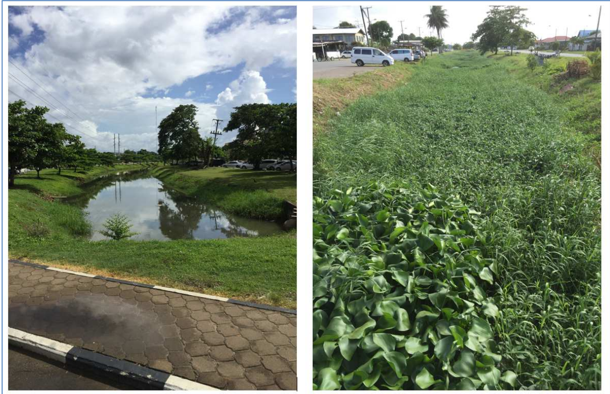
Figure 3-9. Maintenance requirements – recently maintained (left), maintenance required (right).
