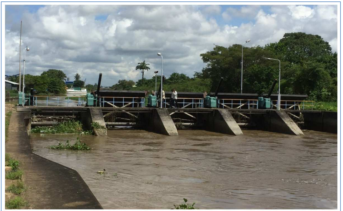
Figure 3-7. Sluice gates at eastern end of Saramacca Canal.
