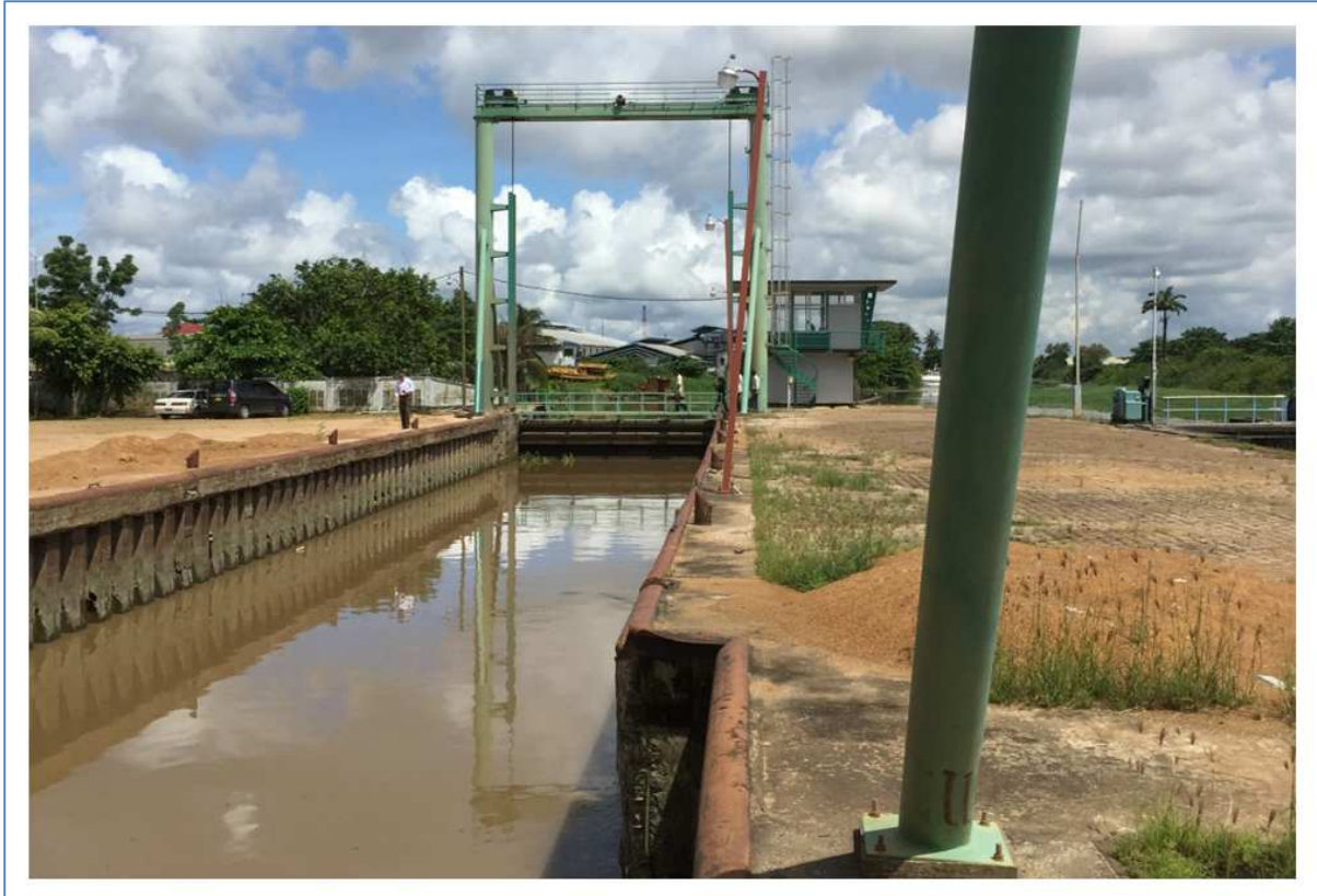
Figure 3-6. Navigation lock on eastern end of Saramacca Canal.
