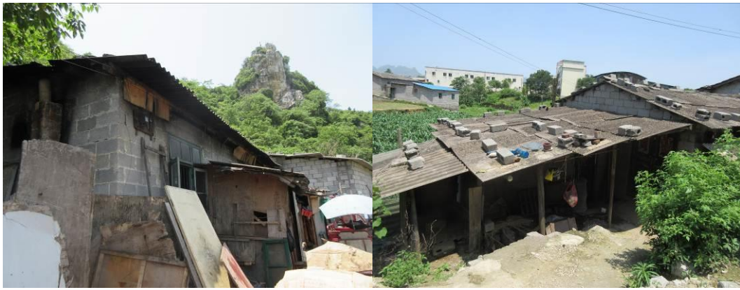
Figure 2-4 Field Attendance Houses to be Demolished
