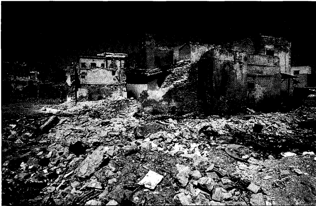
Dilapidated and demolished buildings in Hafsia, before project.
