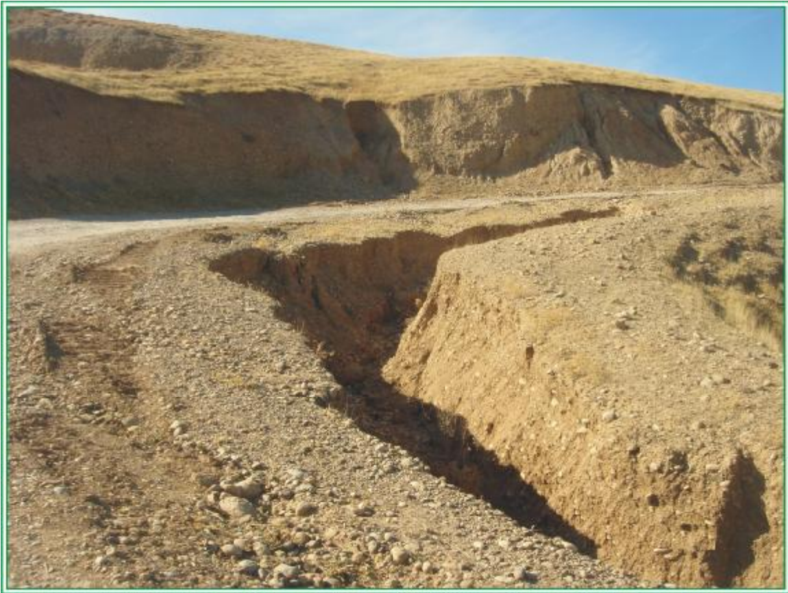
Figure 1.5. The blocked out existing road during the wet period.
