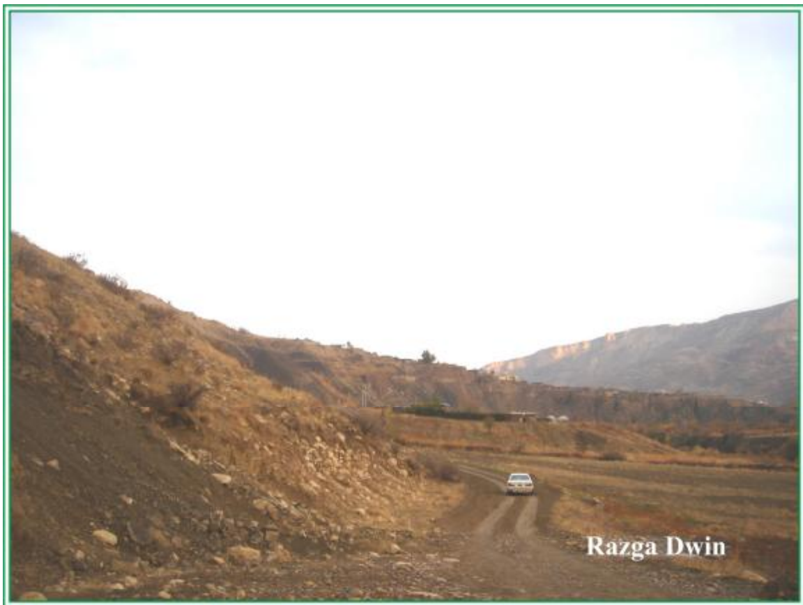
Figure 2.1. The emergency road is blocked out occasionally in winter time.
