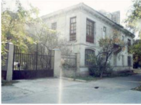
Unreinforced Masonry Buildings with Wooden Floors (URM1)
