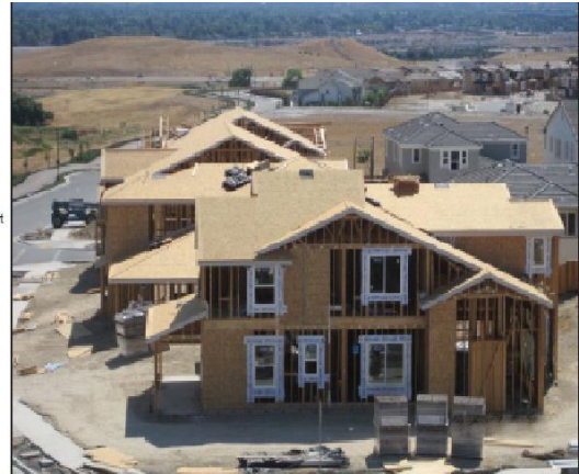
Figure 55 Example of timber frame construction with nailed plywood shear walls for residential buildings (NIST, 2014).
