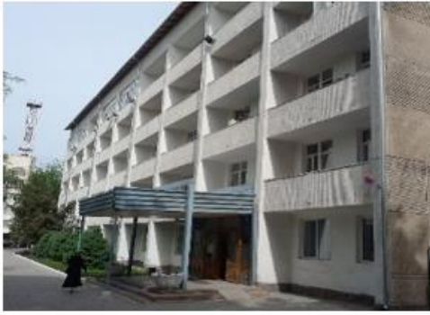
Pre-cast Concrete with Large Precast Panels and Monolithic Concrete Joints Buildings (RCPC1)
