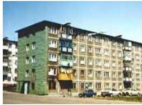
Pre-cast Concrete with Large Panels and Welded Plate Connection Buildings (RCPC2)
