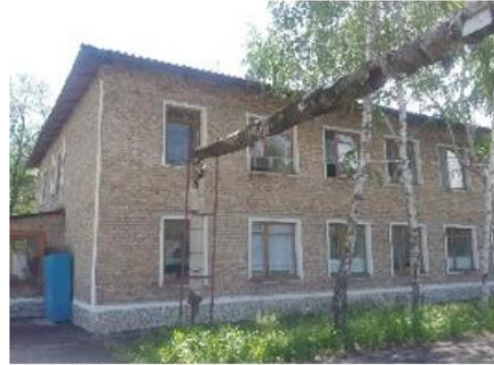
Unreinforced Masonry Buildings with Reinforced Concrete Floors (URM2)
