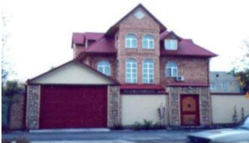
Confined Masonry Buildings (RM1)
