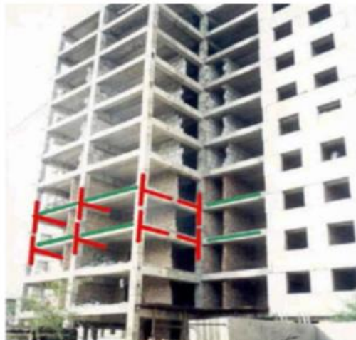
Pre-fabricated Reinforced Concrete Moment Frame Buildings (RCPC4)
