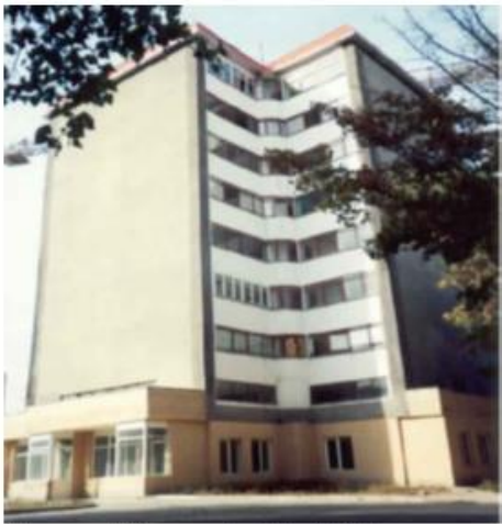
Pre-cast Concrete Flat Slab Buildings (RCPC3)
