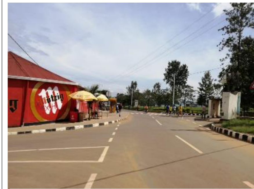
Affected Business premises and University Gate
