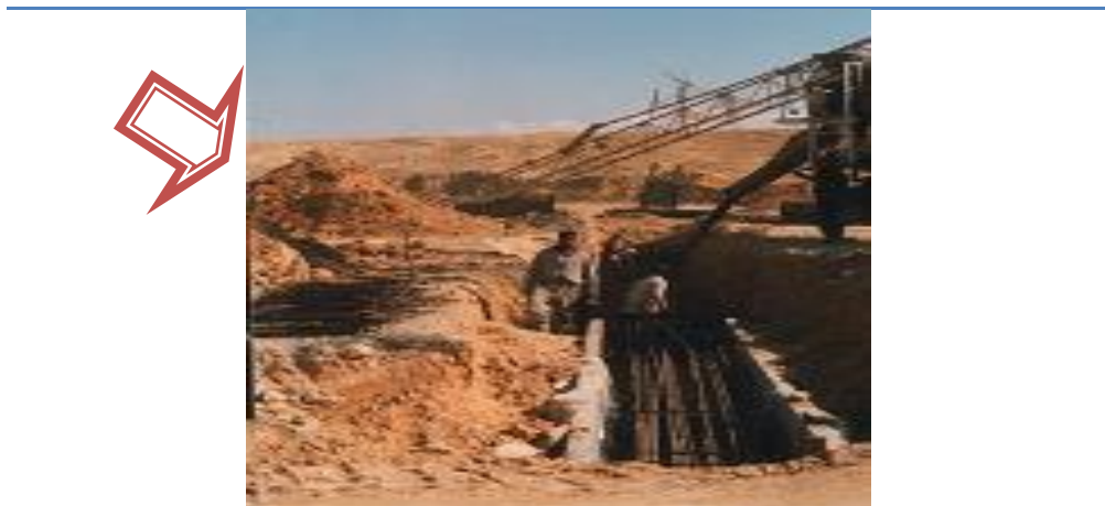
Figure 7: Digging waste and equipments
