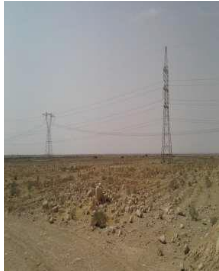
Figure 5-17: Grid connection to the substation
