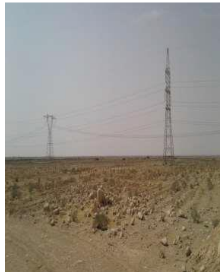
Figure 3-6: Grid connection to the substation
