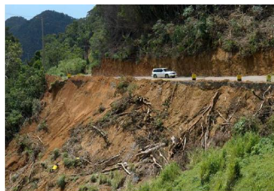
Major landslide on Imperial Highway
