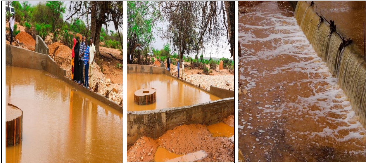
Pictures of Xamxamaa sub-surface Dam in Nugaal Region, After Completion & received rains
