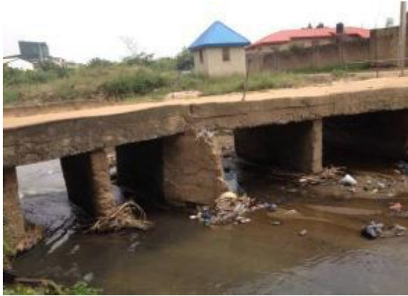
Upstream towards crossing
