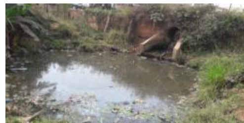
PIC 2.1: Damaged culvert with Inadequate Capacity to discharge flood water
