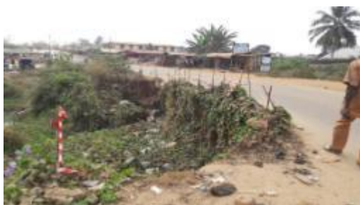
PIC 2.1: Damaged culvert with Inadequate Capacity to discharge flood water
