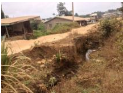
Collapsed culvert
