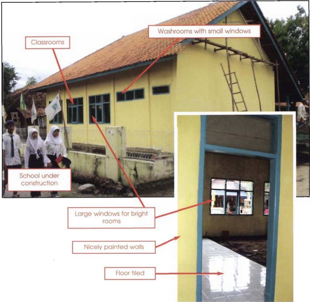
Well-built school building
