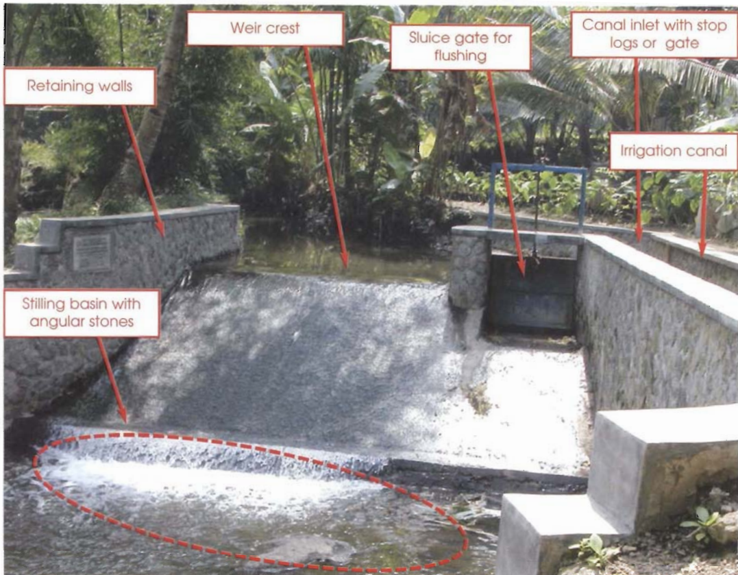
General arrangement of an irrigation weir
