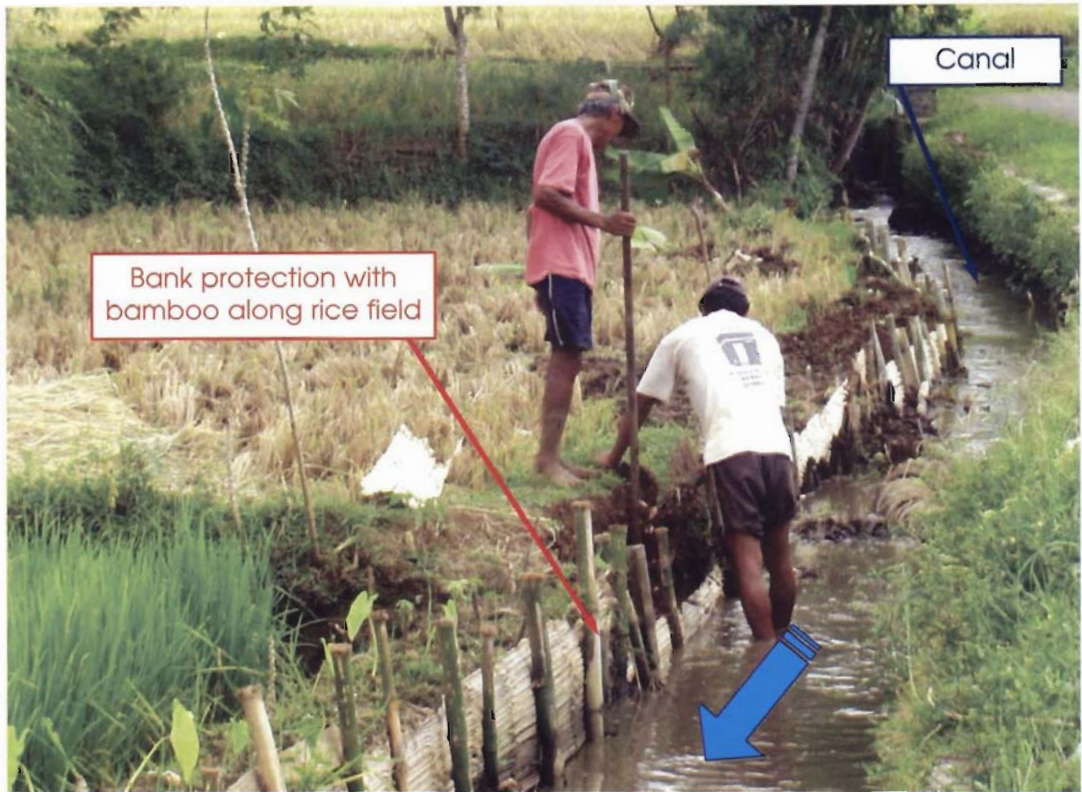
Canal bank protections with bamboo
