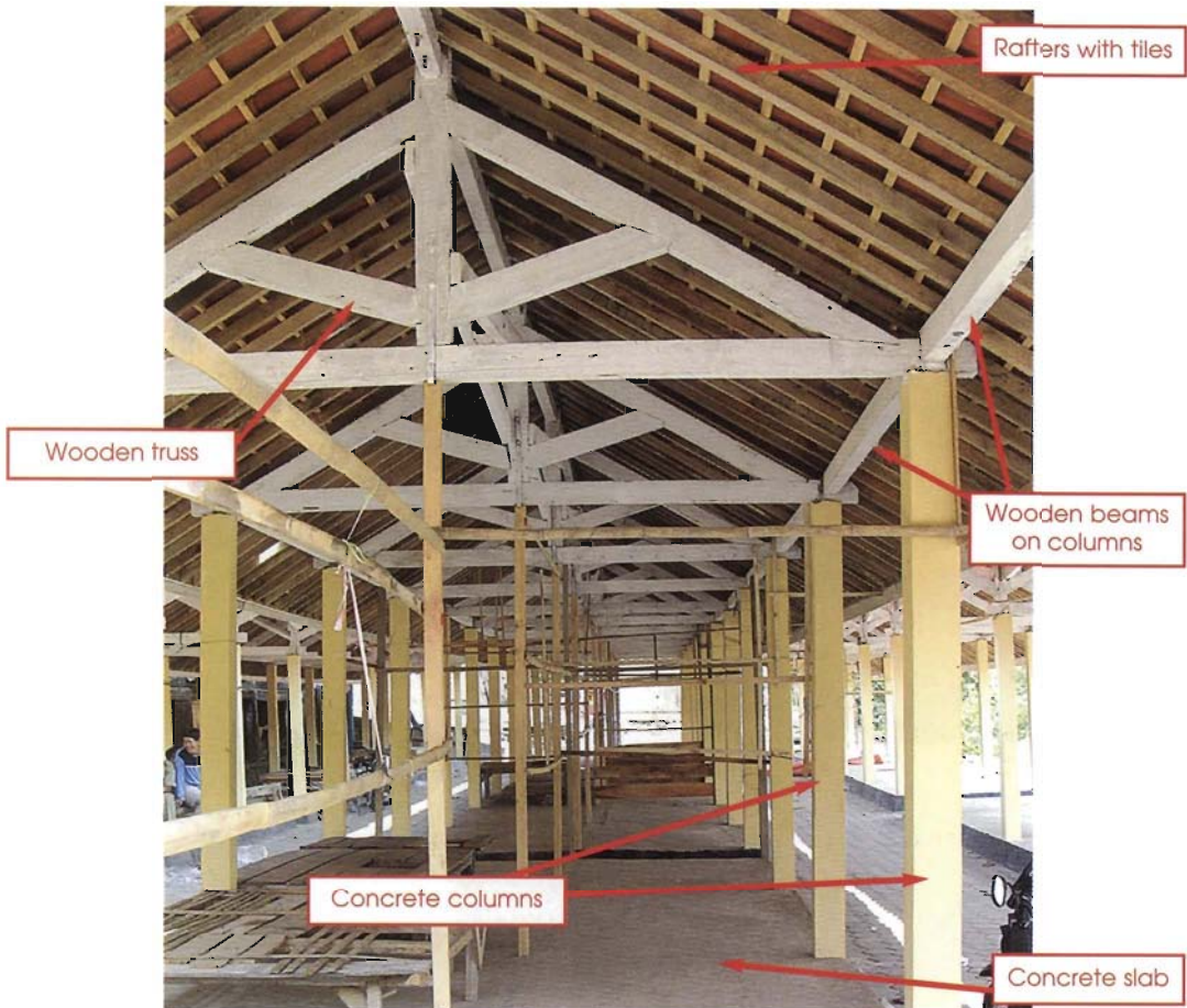
Market shed Type 2: Concrete columns, wooden roof structure and roofing tiles
