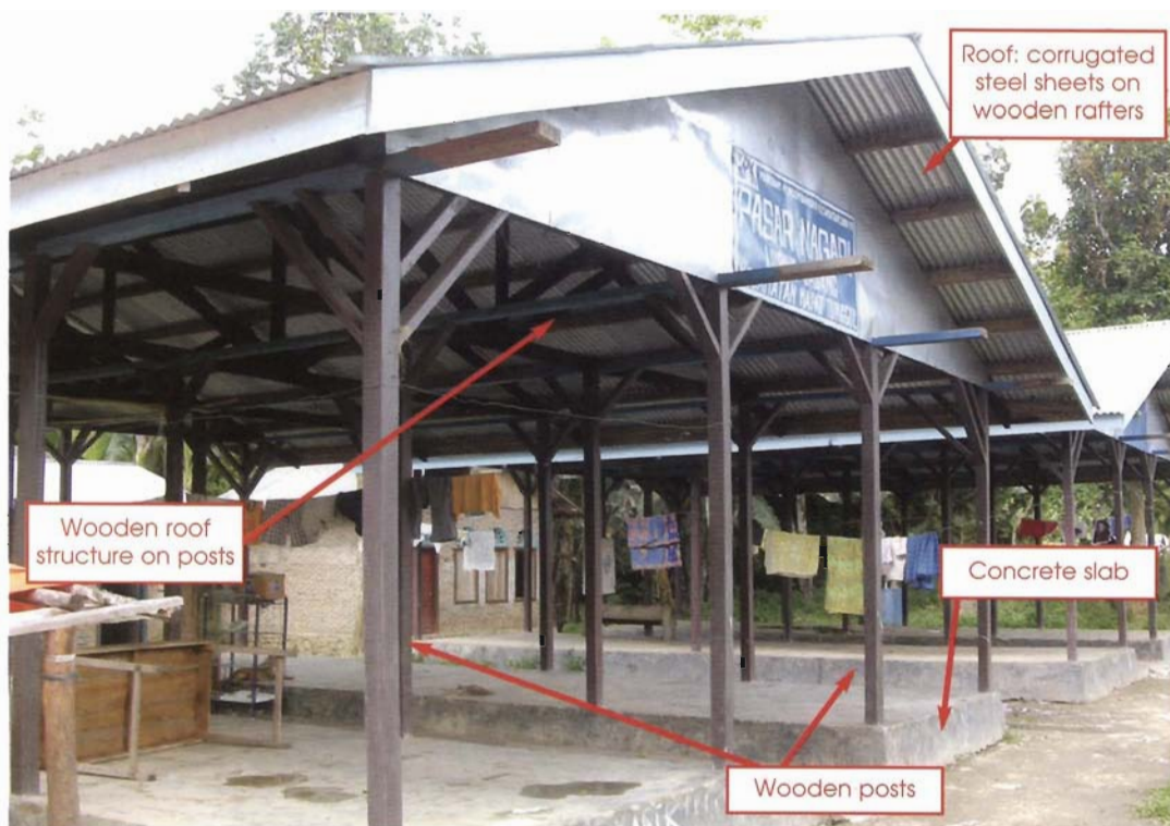
Market sheds Type 1: Concrete slab, wooden superstructure and metal roof
