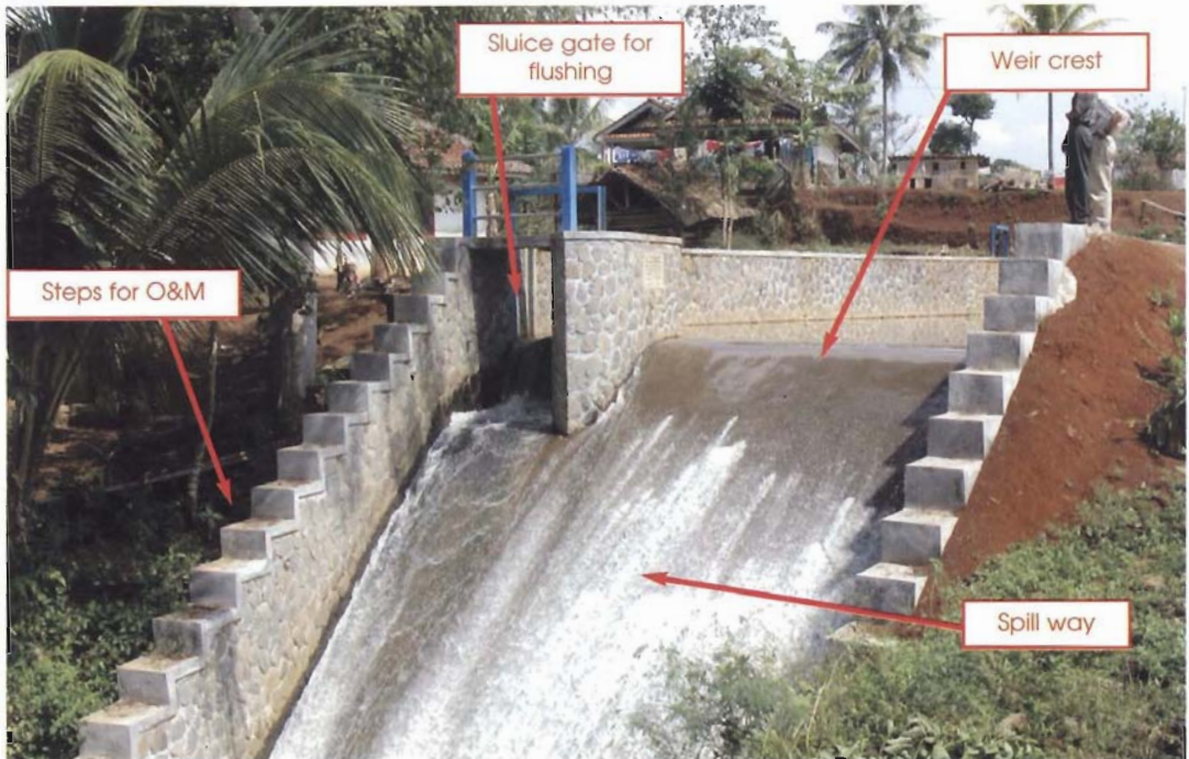
A long spillway of an irrigation weir
