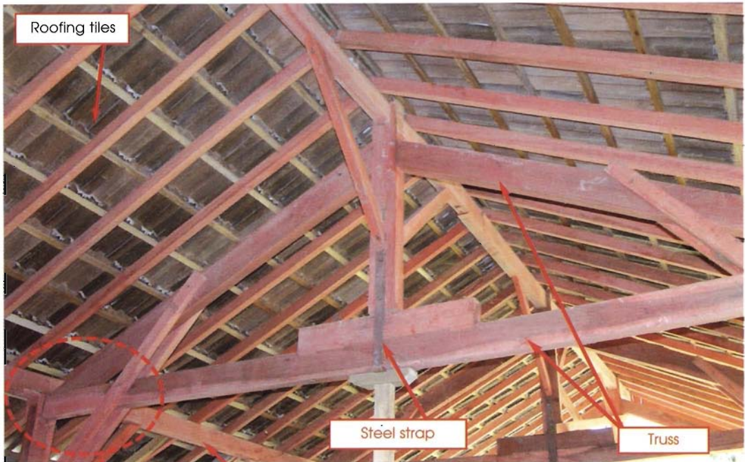
Beam Wooden roof truss on wooden posts
