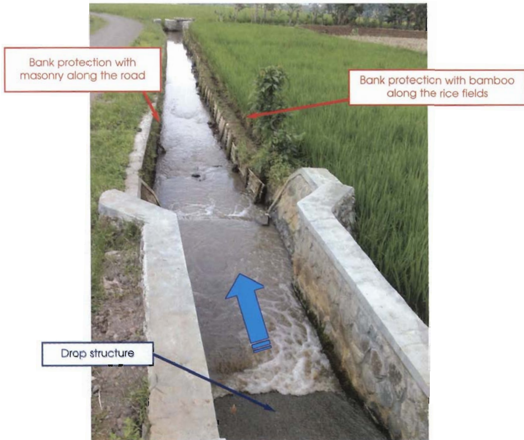
Canal bank and bed protection
