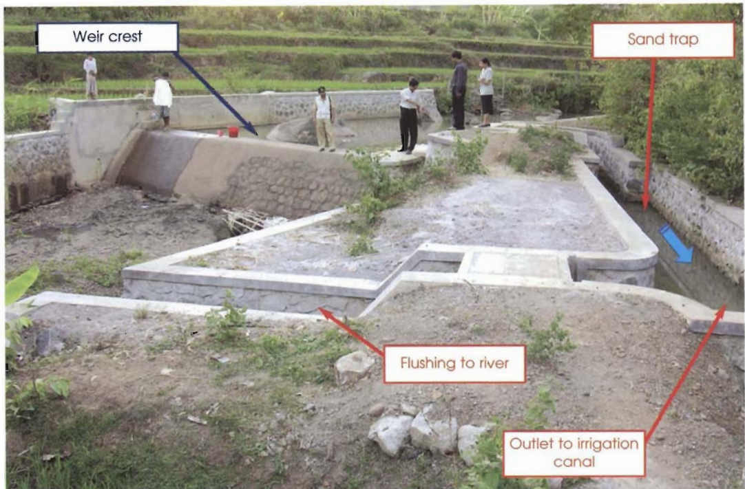
Sand trap integrated in the weir structure
