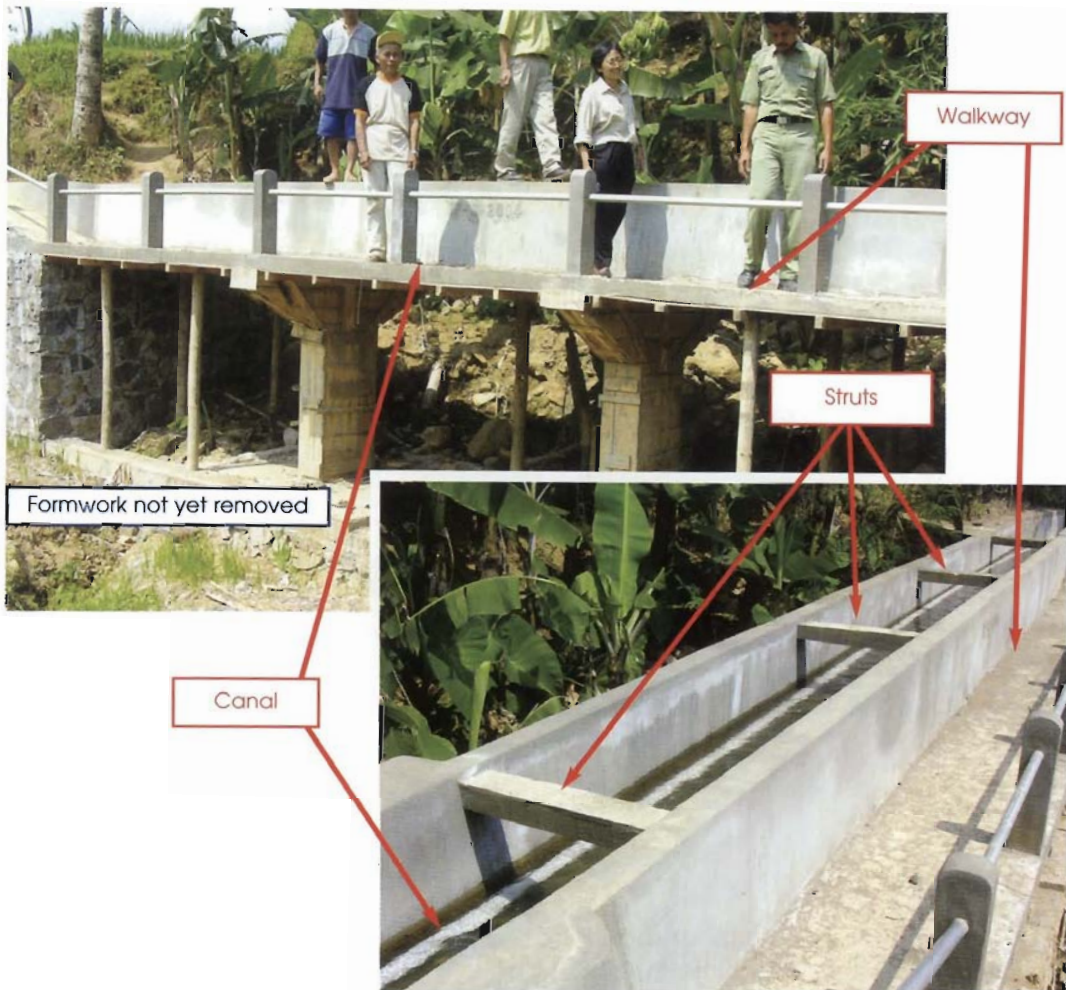
Irrigation canal bridge over a small valley
