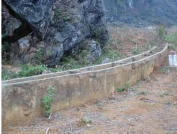
FIGURE 20. SMALL-SCALE IRRIGATION UPGRADE PROJECT IN HA GIANG
