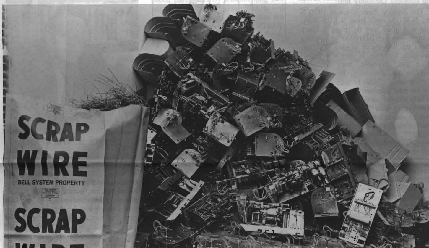
Old telephone equipment being readied for removal.
