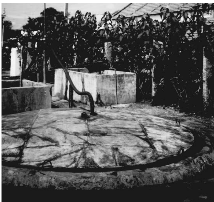
Community biogas digester providing methane to run an electricity generator for lighting and water supply in a village near Bangalore, India.
