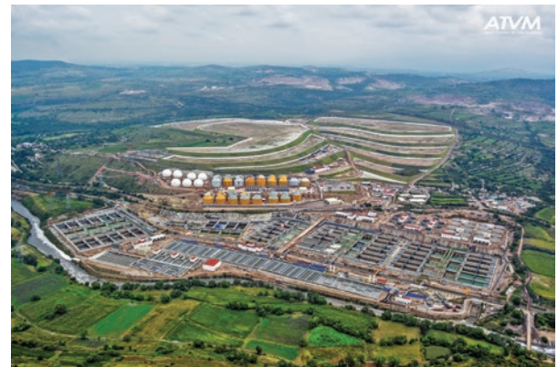
PHOTO 1. Aerial View of Atotonilco Waste Water Treatment Plant
