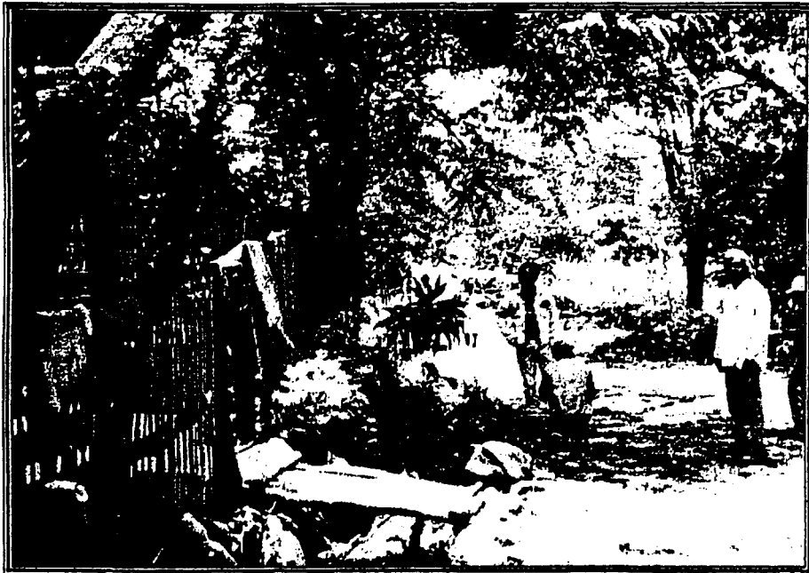
Affected Bamboo Fence at Right Side (Inner Lane) due to widening
