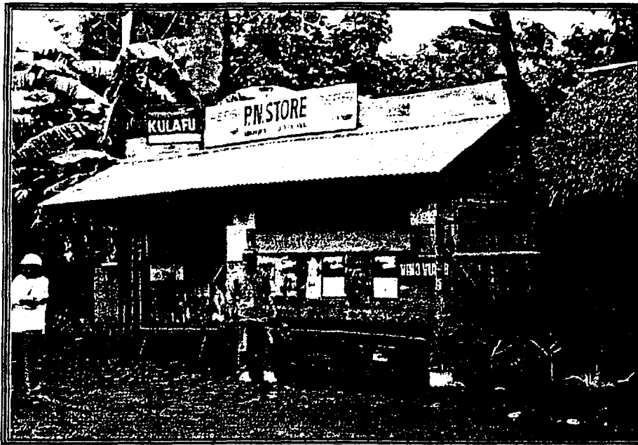
Affected Store, 4.00 m from C/L, Right Side, Sta 86 + 734.00
