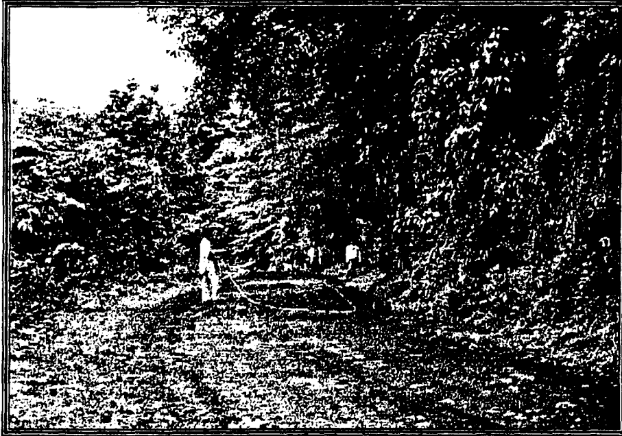
Side Cut (Solid Hard Rock), 1.50 m \approx 3.00 m from C/L, Left Side, Sta 81 + 304.00 to Sta 81 + 445.00
