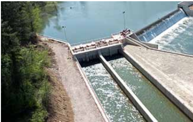
Figure 4-7: Diversion weir
