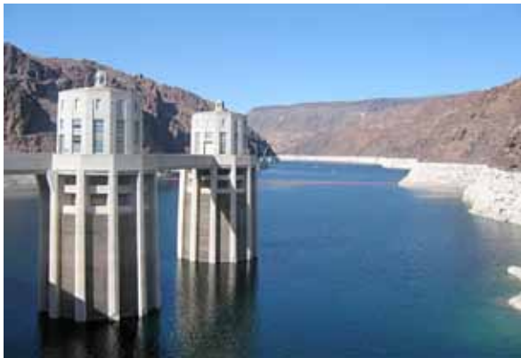
Figure 4-12: Intake tower in reservoir created by the Boulder dam, Colorado, USA
