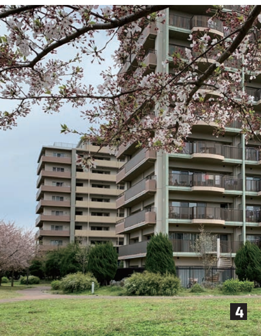
Figure A18.1: Overall View of the Site
