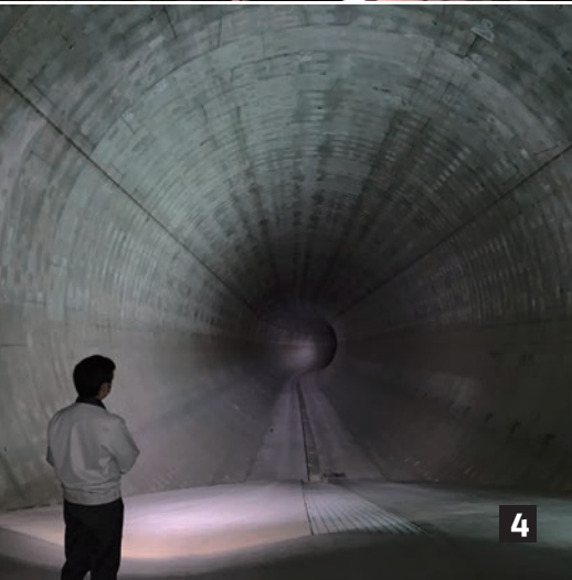
Figure A3.1: Overall View of the Site
