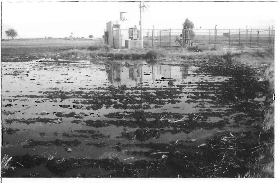
b) inadequately sized and protected wellhead operational zone threatened by agricultural irrigation with urban wastewater
