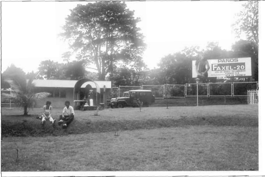
a) well-designed, drained, and maintained wellhead operational zone in rural wooded area
