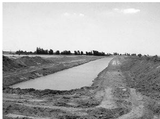
New open drain under construction in Nubariya.
