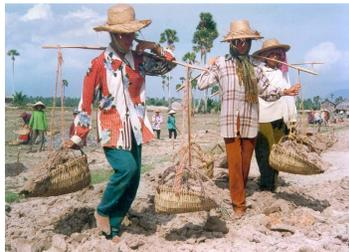
Using labor-based methods, the labor content in road construction and improvement costs is typically in the range 30 to 50 percent of construction cost. For maintenance work the percentage labor cost can be in the range 50 to 80 percent. Corresponding percentages for equipment based work are 10 percent or less.
