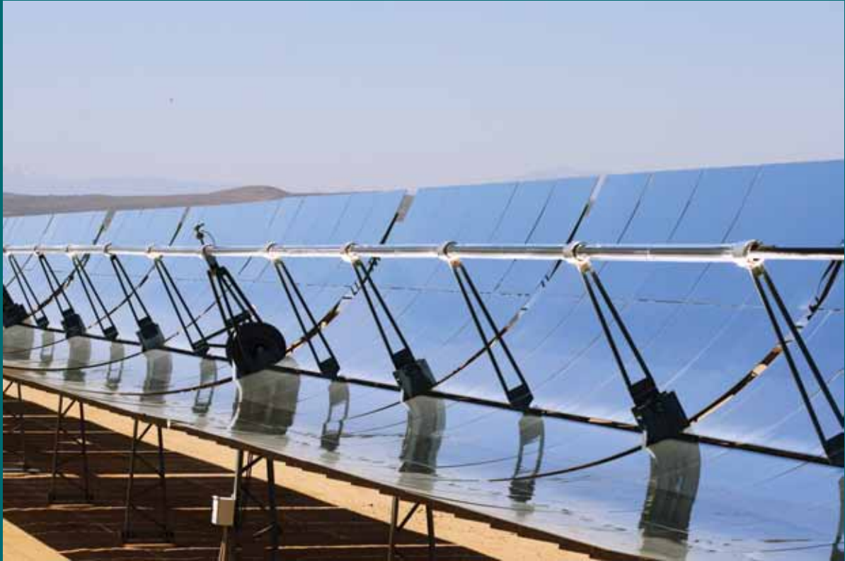
Figure 7: An Example of a Parabolic Trough Concentrator
