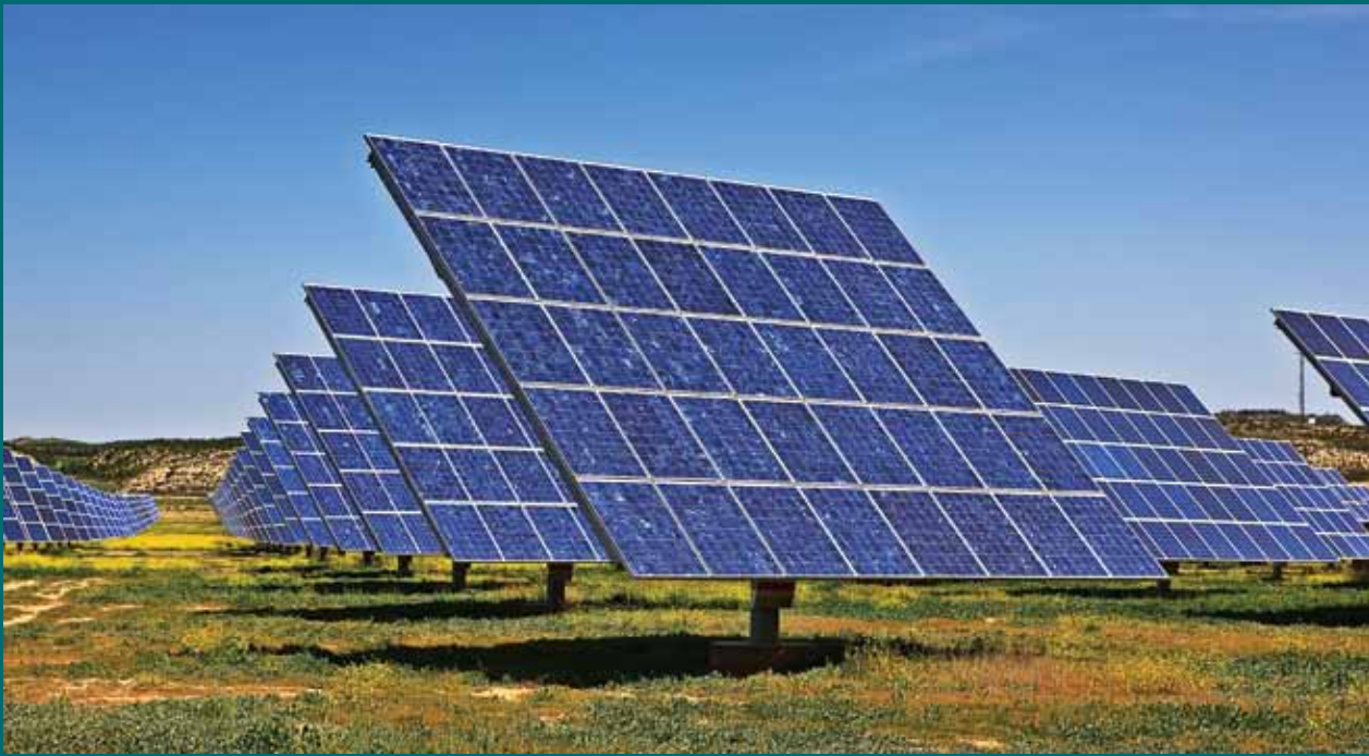
Figure 5: An Example of a Tracking PV Plant
