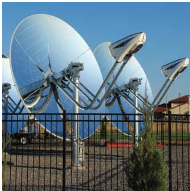
Figure 13: An Example of a Parabolic Dish System
