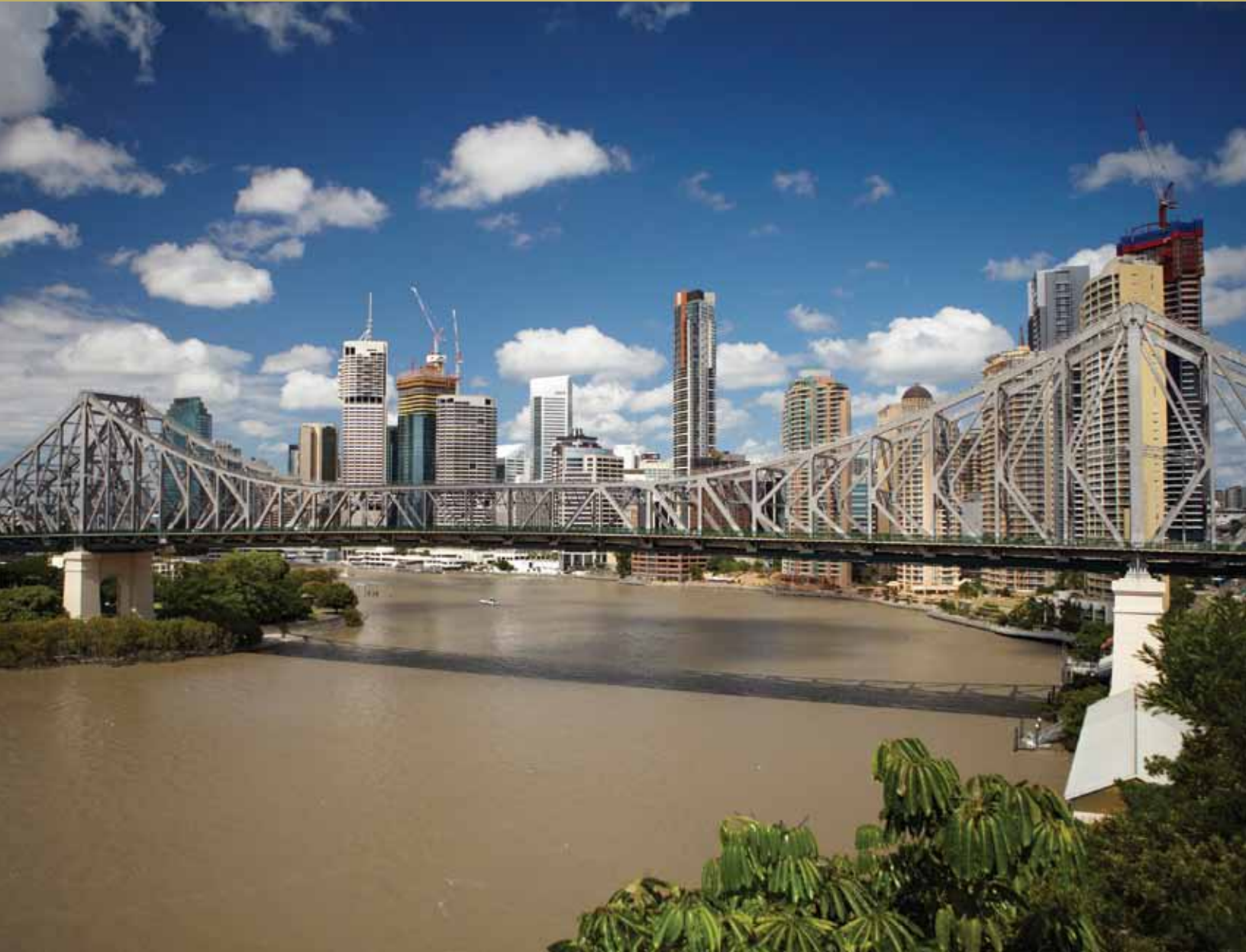
Aerial Story Bridge post flood. Photo courtesy Brisbane Marketing.
