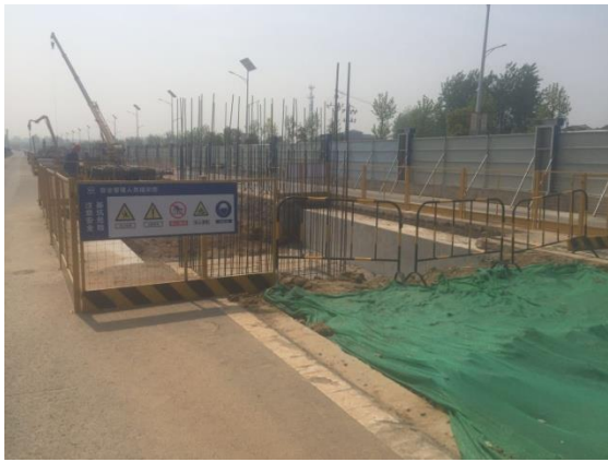
Construction foundation pit
