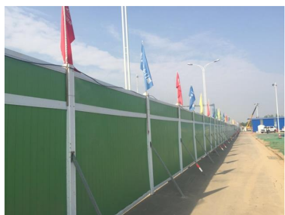
Construction site fence
