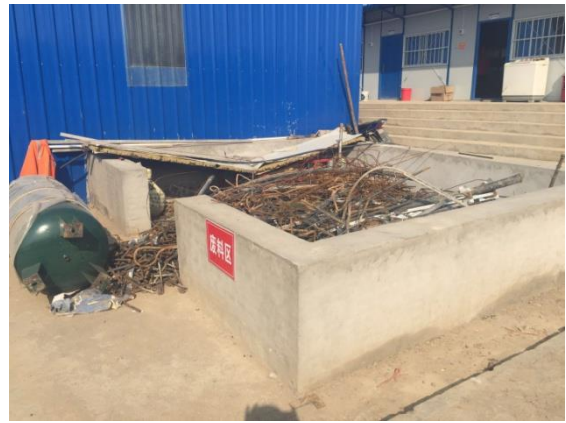
Construction waste stacking area
