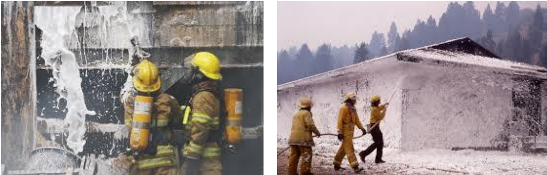
Figure 7.7: Application of Class A foam on a structure during a wildfire (on the left picture) and application of foam using CAFS system in a structure protection configuration (on the right picture)
