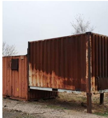
Training facilities for work with toxic gases in FRS ID71 Yerevan
