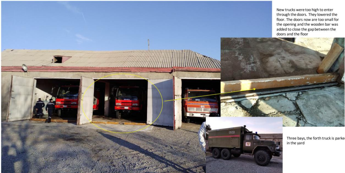
Figure 5.14: Two brand new mid-size ISUZU fire tenders housed in a degraded FRS building which floor needed to be lowered in order the be able to accommodate the new vehicles – example from FRS ID9 in Gyumri, Akhuryan.
