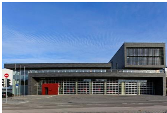
FRS with 4000 m2 - 8 bays for fire engines + 2 bays for maintenance, Vilnius, Lithuania Source:
