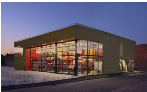
FRS for 3 fire engines, Vleuten, The Netherlands
