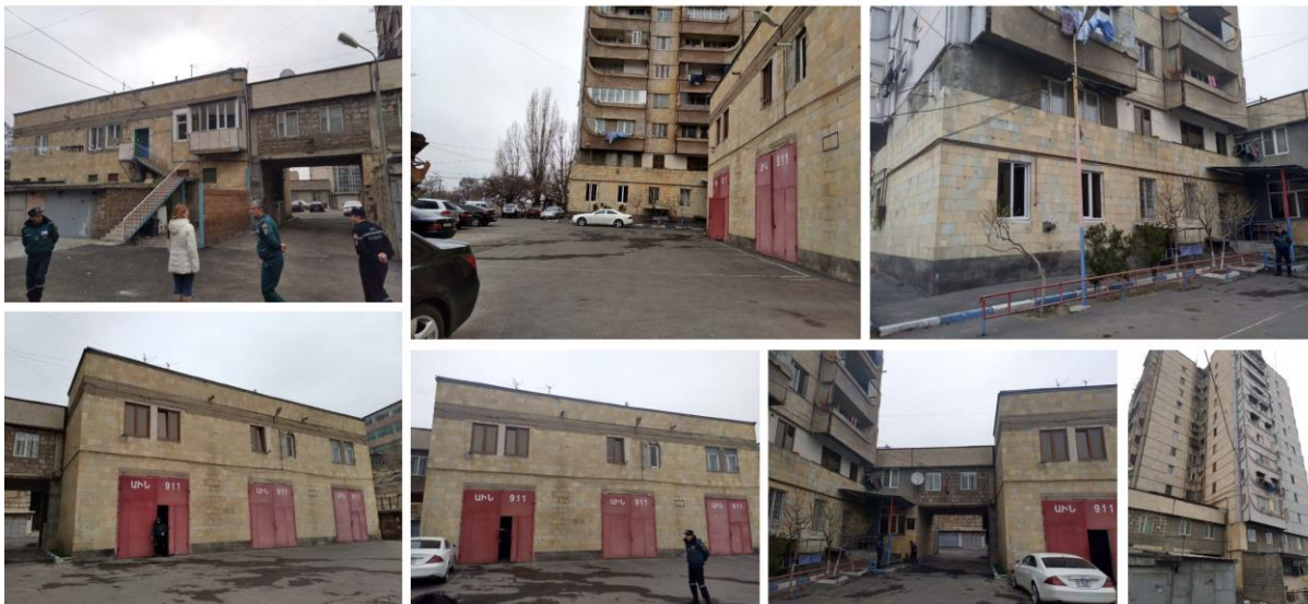
Figure 5.22: FRS which is partially located on the 2 nd floor of a 13 storeys high residential building connected to the apparatus bays via a bridge – FRS ID61 in Yerevan.
