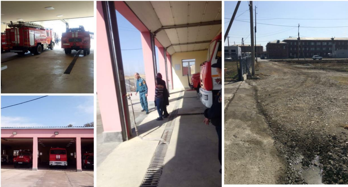
Figure 5.18: Recently renovated FRS with improved conditions in the garage by installing modern automatic doors, drainage and fume gas extraction system equipped with aged fire engines – example from FRS ID43 in Artashat.
