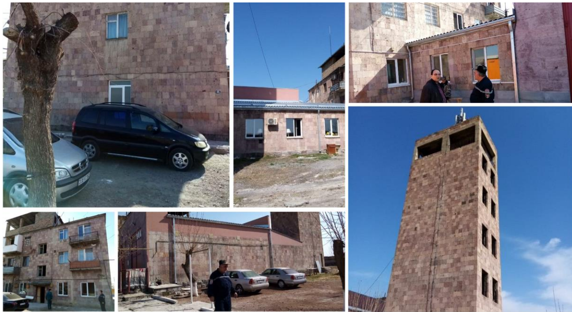
Figure 5.21: FRS sharing part of its first floor with a 3 storey high multifamily residential building – FRS ID44 in Masis.
