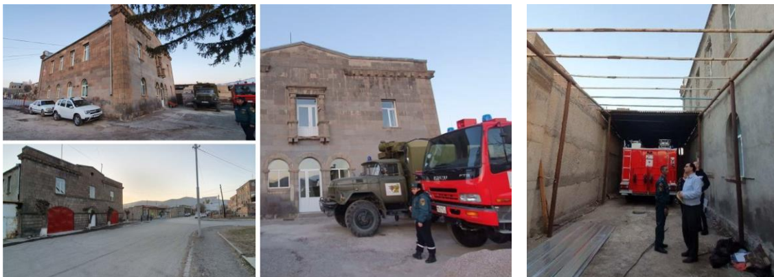
Figure 5.17: Brand new mid-size fire tenders which cannot fit into the FRS garage and stay outside – example from FRS ID57 in Sisian.
