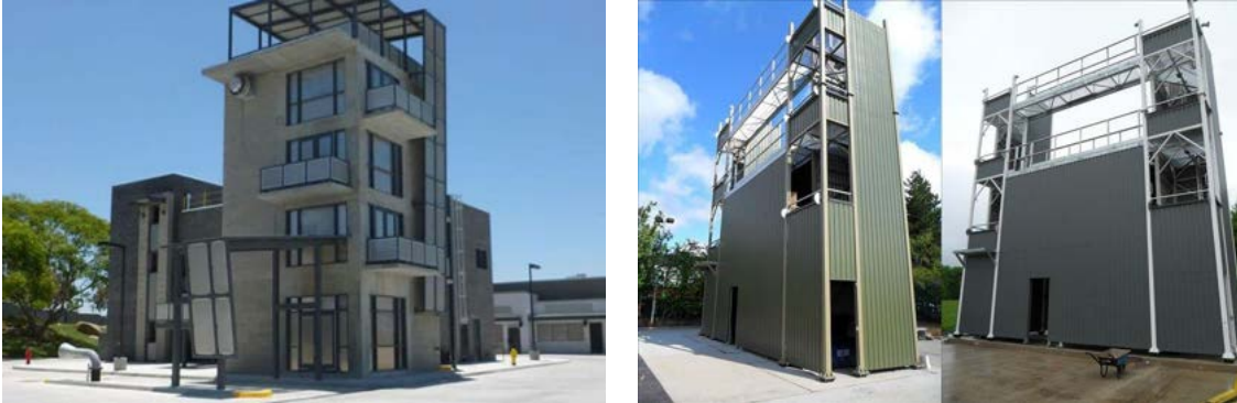
Figure 8.21: Example training towers
