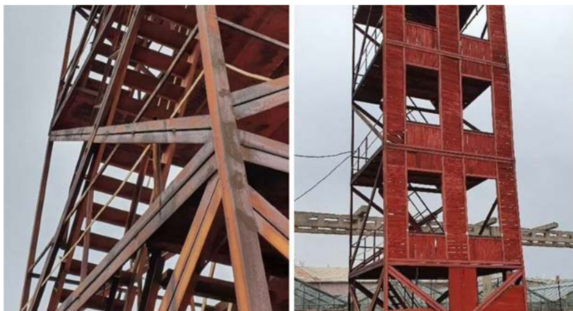
Training tower in FRS ID71 Yerevan
