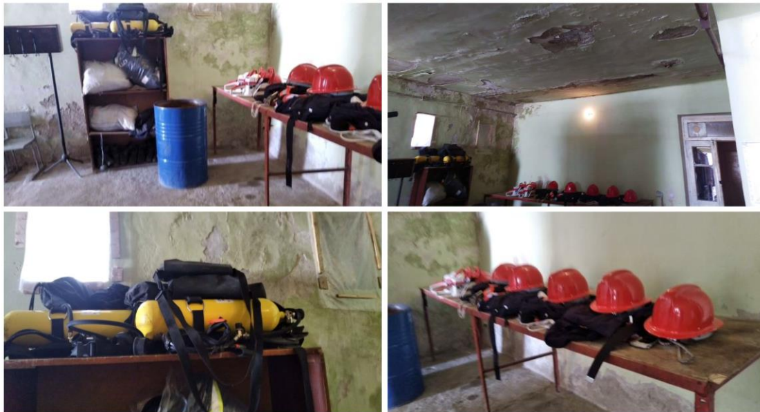
Figure 5.16: New PPE with no space and adequate conditions for proper storage – example from FRS ID11 in Ashotsk.
