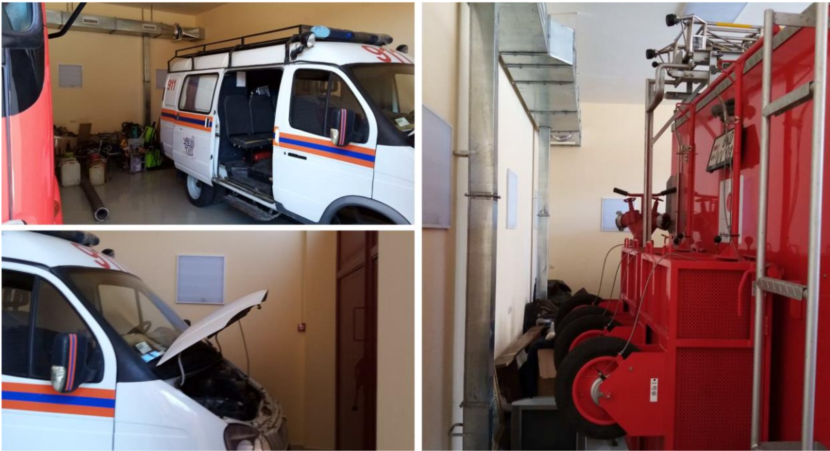
Figure 5.28: Fume gasses exhaust system and epoxy non-slippage cover with a drainage in the garage – examples from Meghri.
