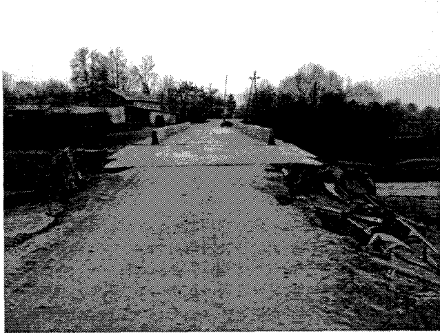
Box 2. Bridge and river bank protection at the Kulyabdarya canal
