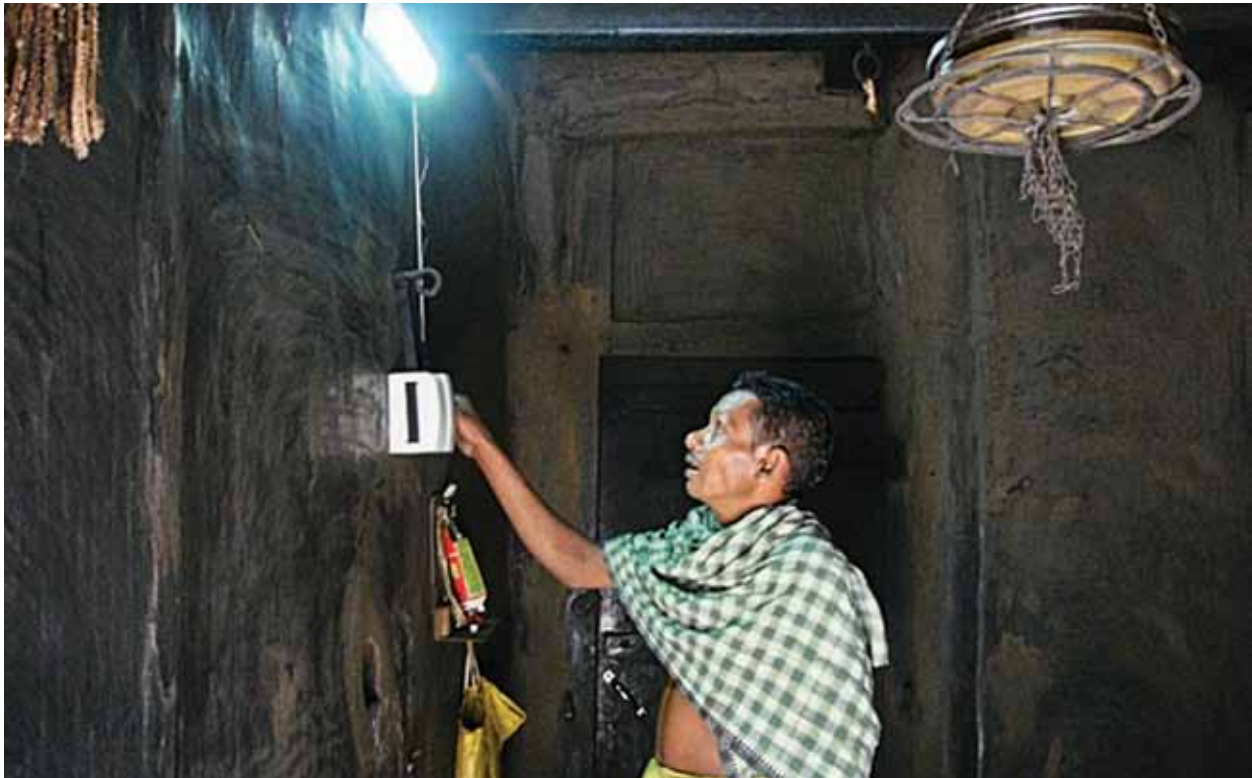
Image courtesy of Schneider Electric
