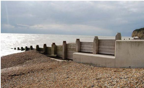
Example of hard engineering solutions, a concrete and wooden groyne, Photo Credit: Nigel Chadwick
