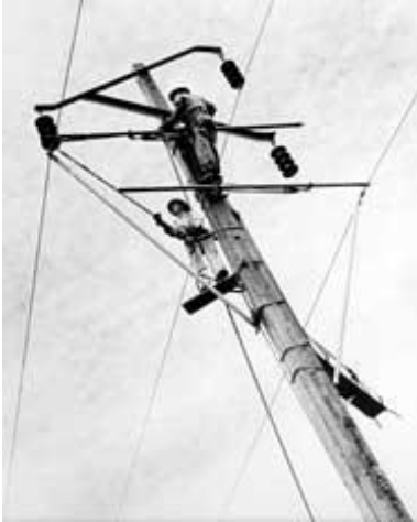
Maintenance workers erecting and connecting 66KV transmission lines to link the Los Cipreses hydroelectric power plant with the Sauzal hydroelectric plant and other substations.
