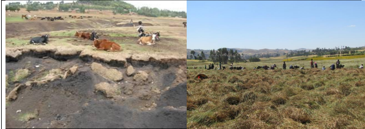
Over-grazing and landslide, before
