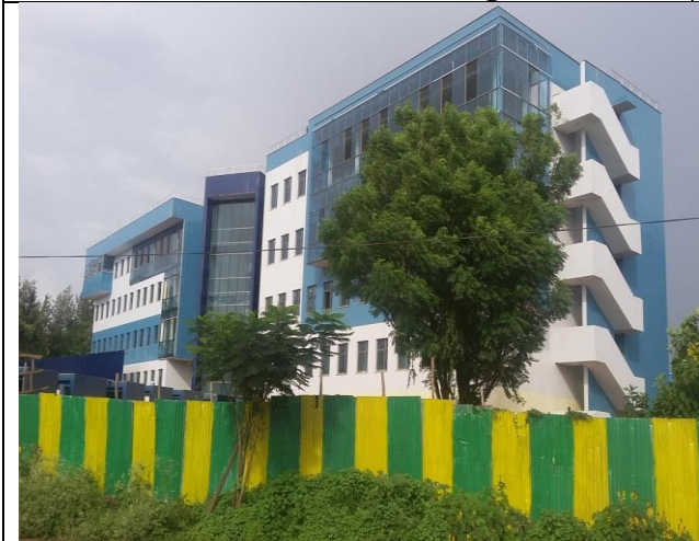
TaSBO office building
