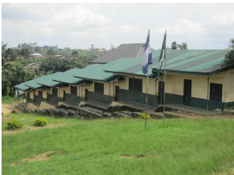
Plate 4.1: A primary school in Ikot Anwatim gully complex area
