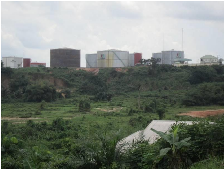
Plate 3.1: NNPC petroleum products storage depot (background) and lower watershed of gully complex area (foreground).
