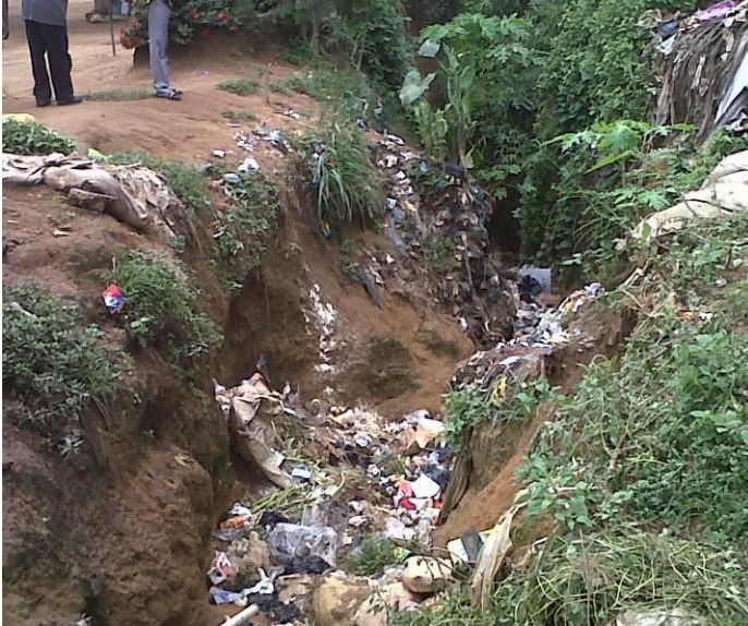
Plate 4.3: Use of gully as a refuse dump in Ikot Anwatim
