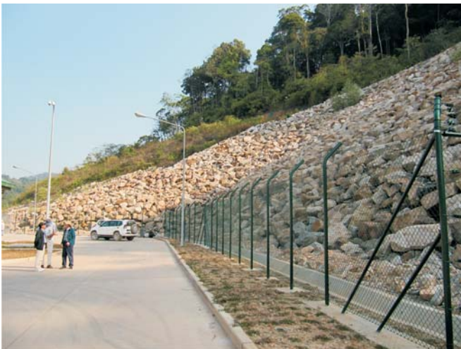
Riprap boulders holding back potential erosion at the dam site.
