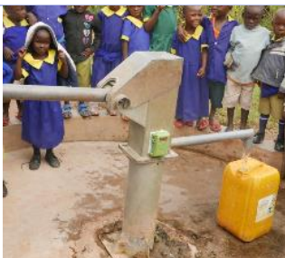
Figure 16: SweetSense Monitoring Unit on an Afridev Handpump (Photos Courtesy of SweetSense)
