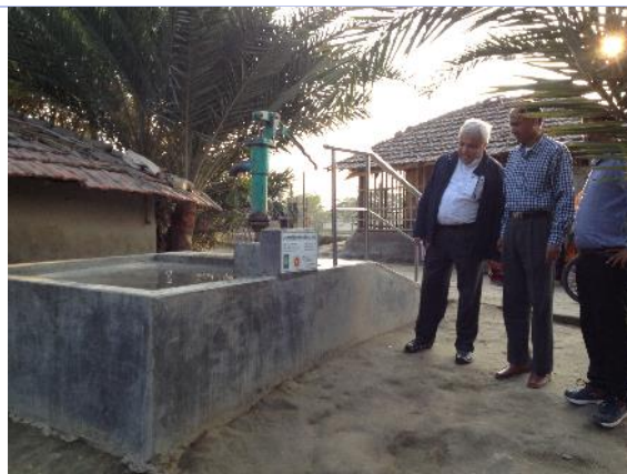
Figure 28: Raised handpump water point with ramp and rail for disabled access (photo: S Furey, HYSAWA Bangladesh 2017)
