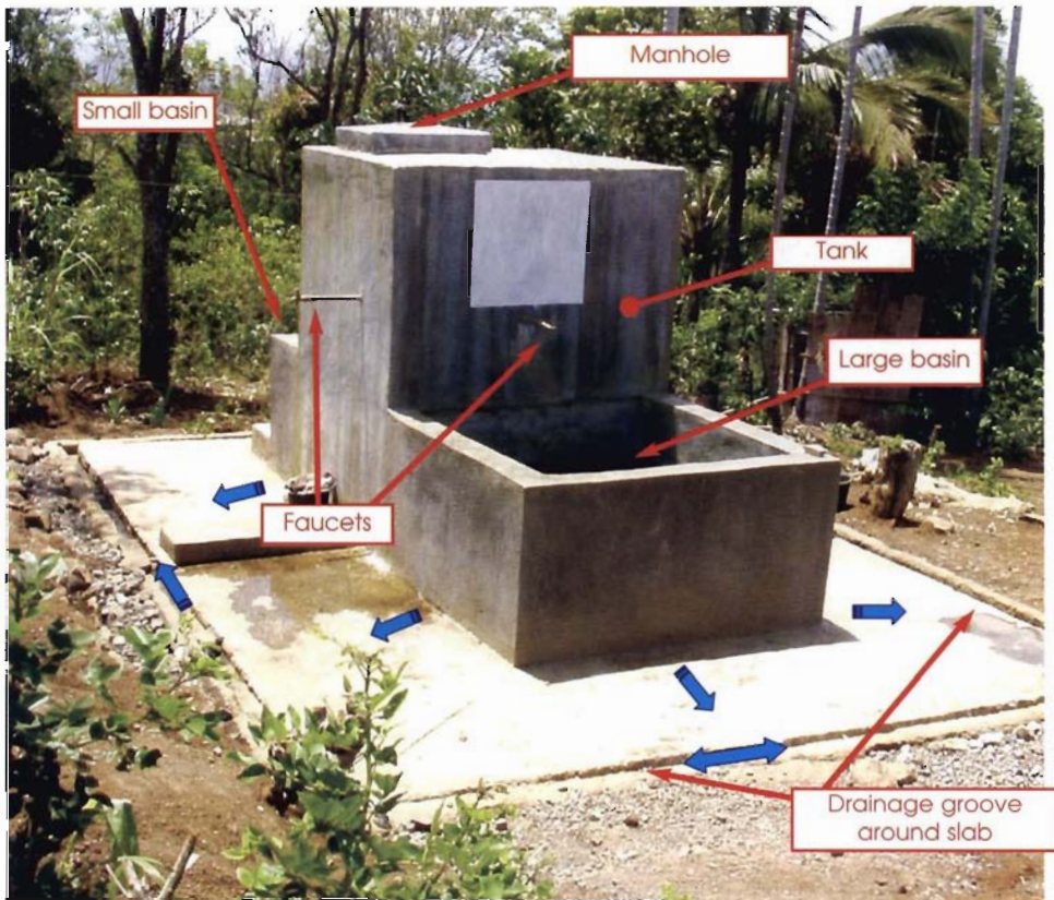
Tank with public hydrant and public washing / laundry place (2 basins)
