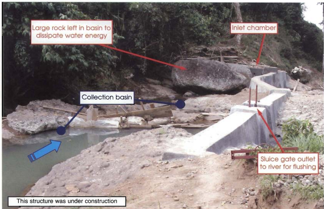
Water intake in a larger river
