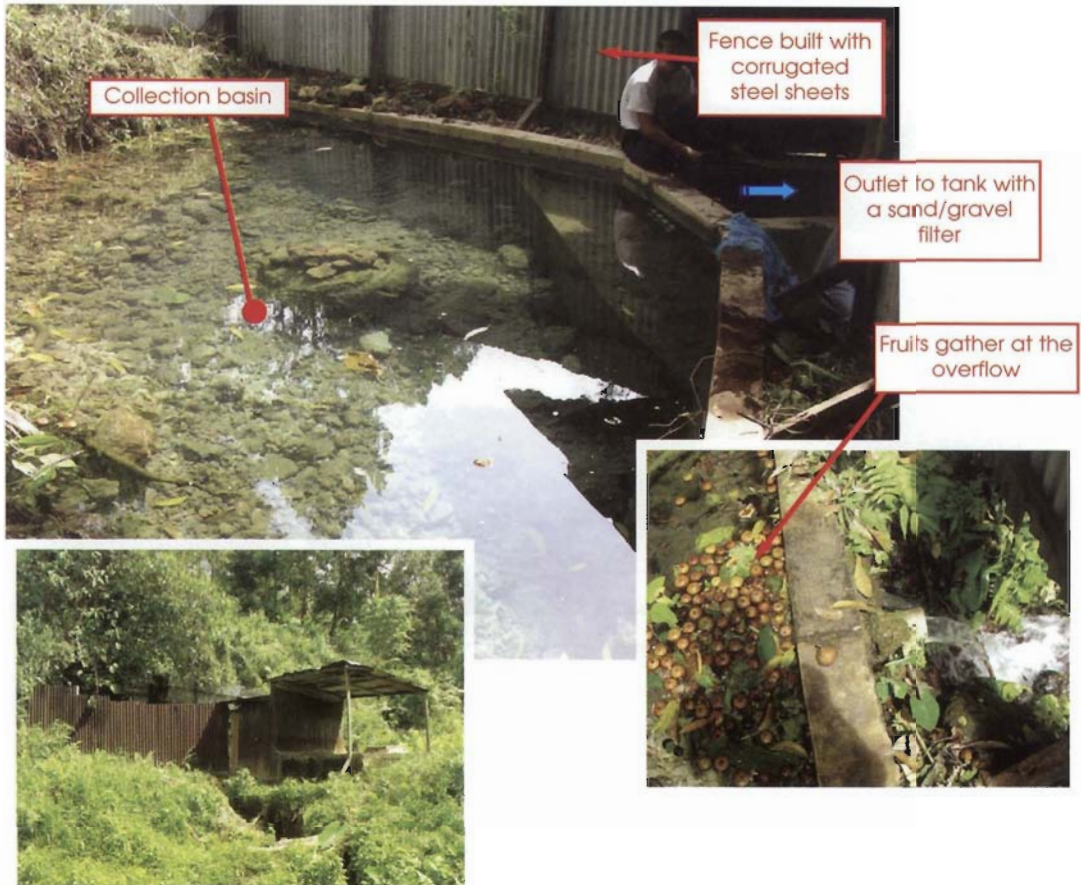
Collection basin for a spring capture
