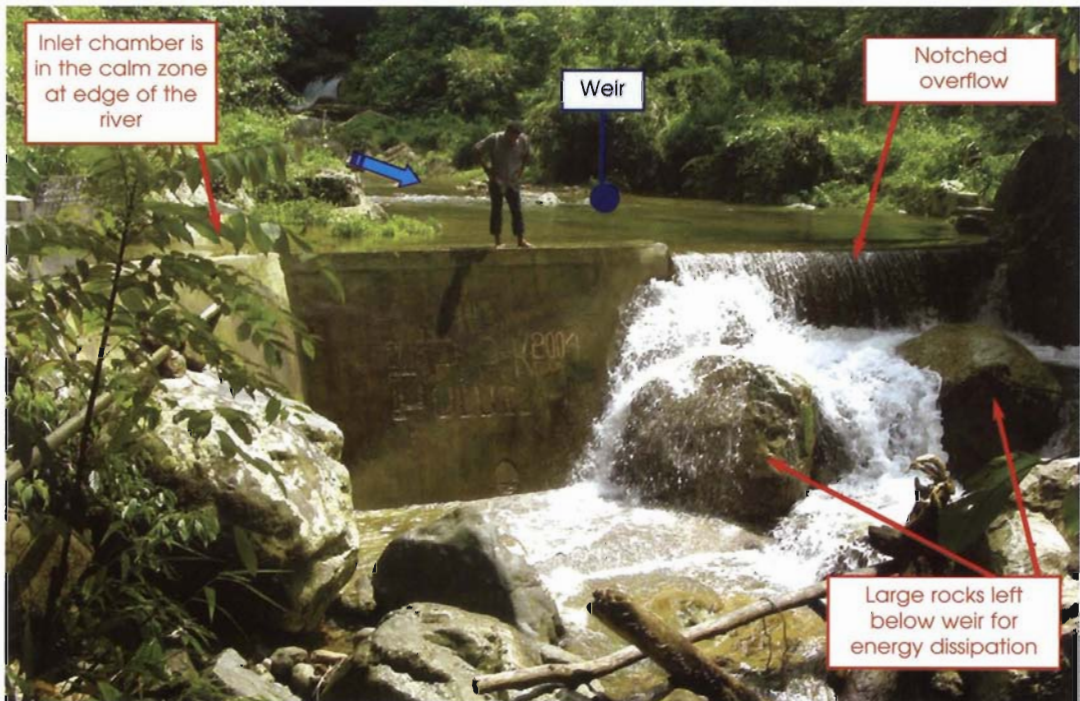
Water intake in a river
