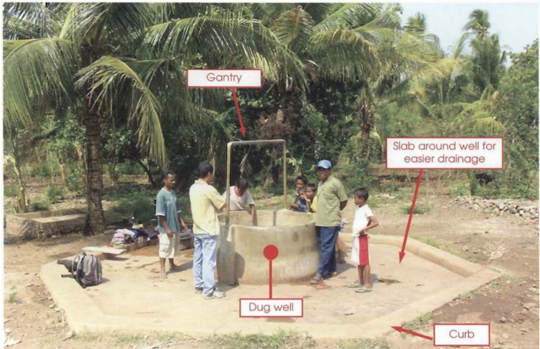
Dug well with all necessary facilities
