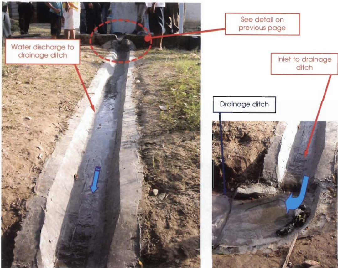
Water discharge to a drainage ditch
