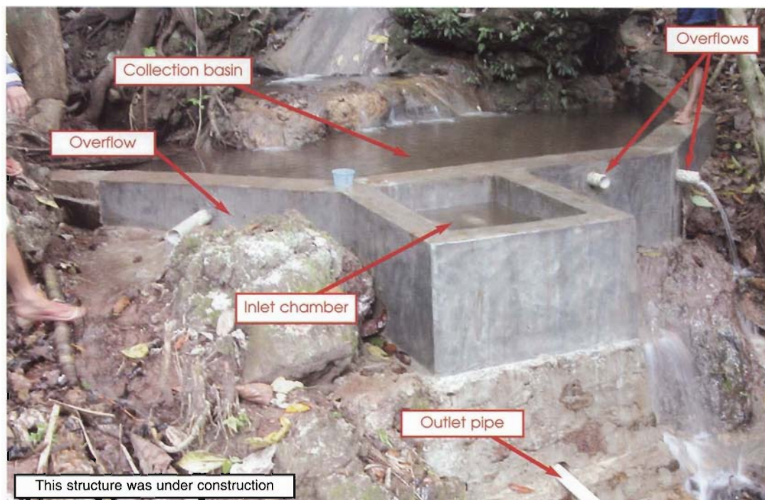
Collection basin in a small stream
