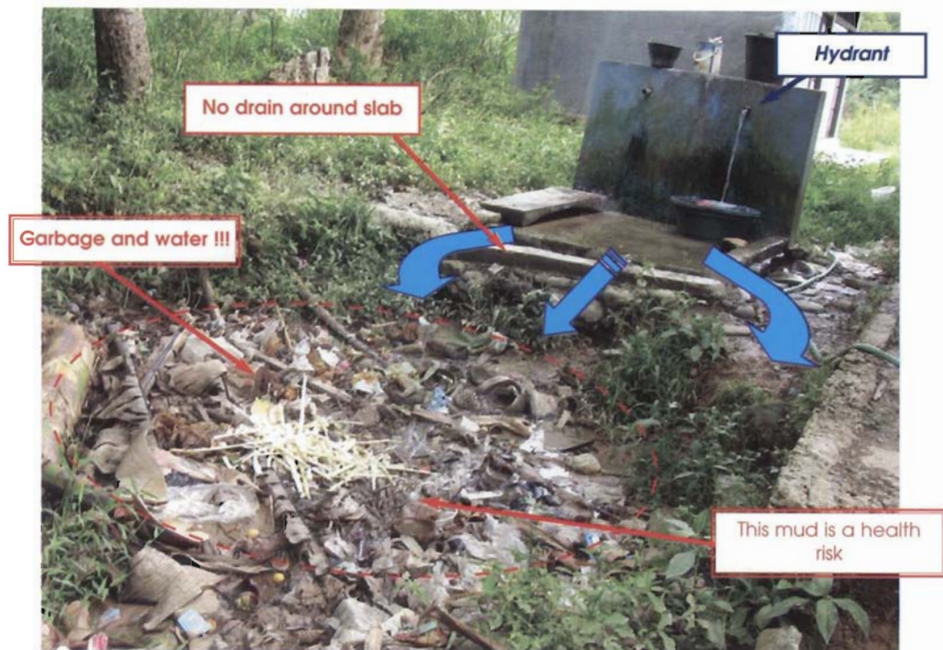
Spilled water flows to a garbage disposal area
