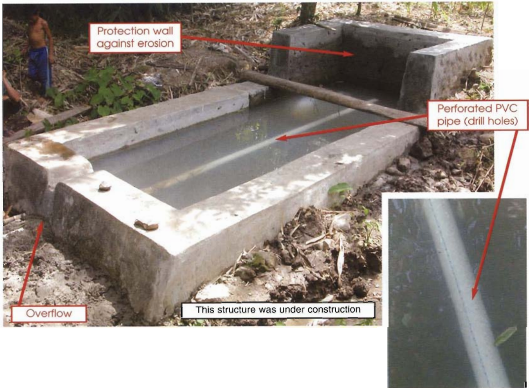
Collection basin for a spring capture
