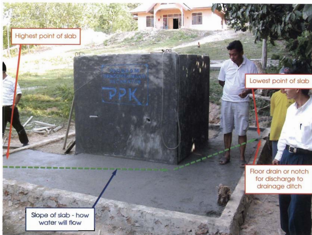
Sloped slab around tank (under construction)
