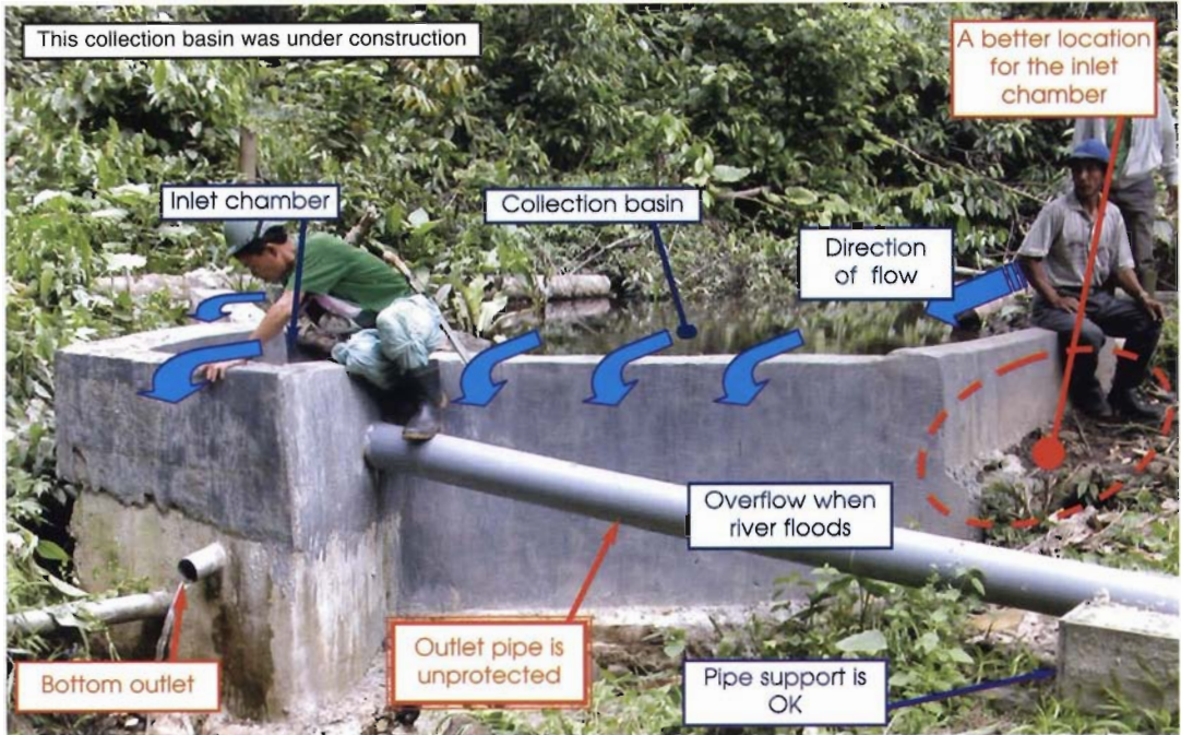
The outlet pipe crosses the flooding zone of the river
