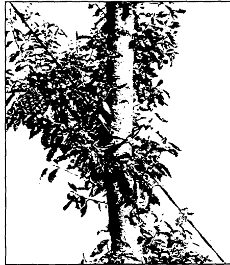
Fig. 52. A living tree is used as a pole and the two-conductor ABC is deadended on both sides of the tree.
