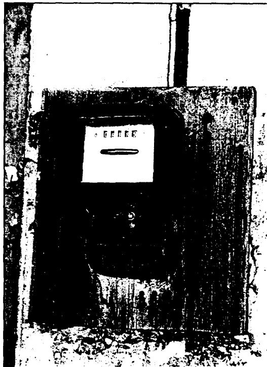
Fig. 111. View of a bottom-connected meter.
