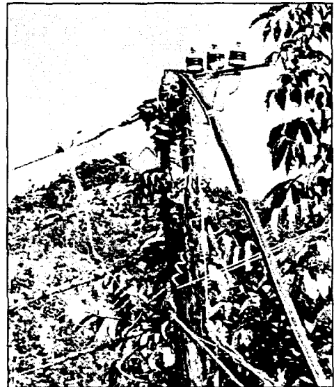
Fig. 97. Three lightning arresters on a three-phase, four-wire line just outside the powerhouse.
